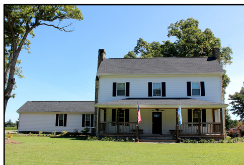
Figure 29: Currin House (VN0387) features replacement siding, windows, doors, and porch.
