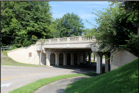
Figure 24: Seaboard Railroad Overpass (VN0201)
