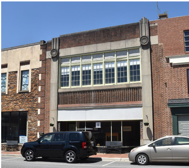
BK0571's concrete pilasters, floral medallions, and brick details are unusually decorative for Valdese's commercial architecture. It also has common characteristics such as its recessed entry and a black tile bulkhead. Photo by author.
