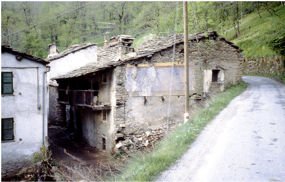
Exposed stone and banked construction as shown on a house in the Waldensian valleys. Photo by Catherine Bishir, June 1985. Burke County Front Matter, Western Regional Office File Room, North Carolina State Historic Preservation Office, Asheville, NC.
