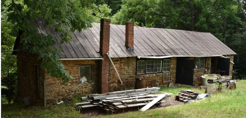
The original John H. Pascal House (at BK0094) is banked into a hillside. It originally consisted of about a third of the current building, which was later extended to the right. Photo by author.
