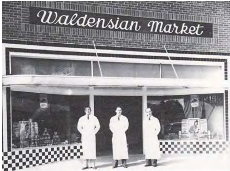
The historic façade of the Waldensian Market (BK0582). Photo from “Then & Now Walking Tour Downtown Valdese.”
