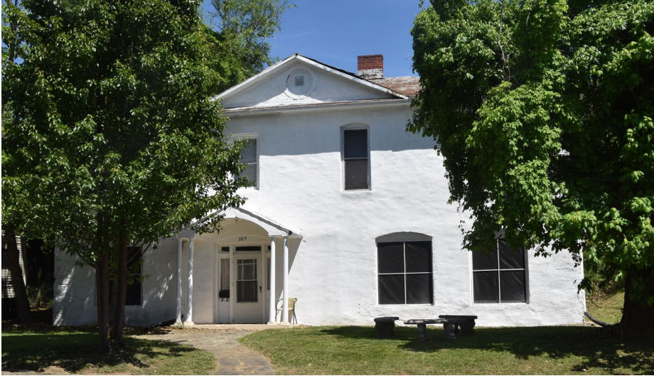
The Sala House (BK0600) exhibits a stucco exterior, reminiscent of “formal”architecture in the Waldensian valleys. Photo by author.
