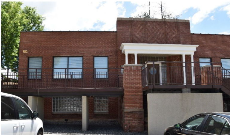
The results of the exterior renovation of the Waldensian Hosiery Mill (BK0284). The concrete wall conceals the original stairs. Photo by author.
