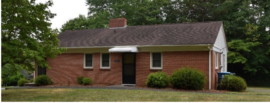
The Pilot Club (BK0526) blends into its surroundings in a residential neighborhood. Photo by author.
