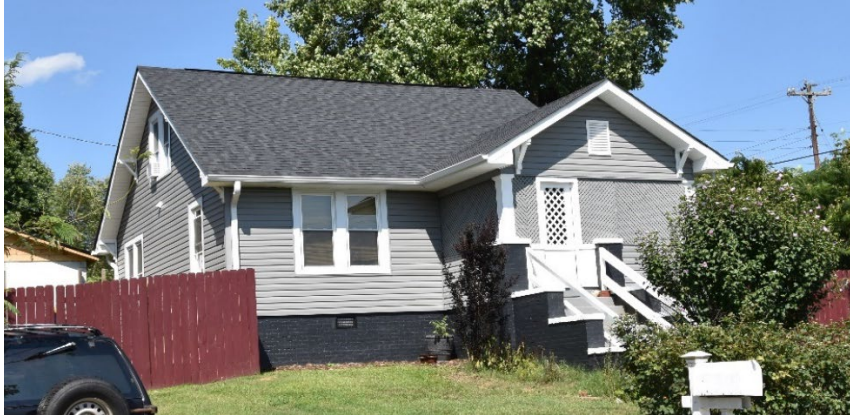
Typical changes to residential buildings in Valdese include enclosed porches, vinyl siding application, and replaced windows. All three can be seen on BK0504. Photo by author.
