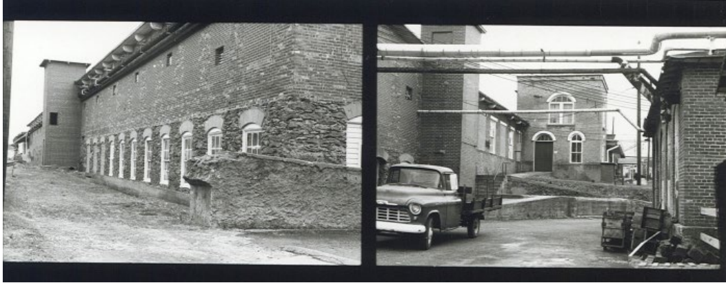
These photos show the Valdese Manufacturing Company before the demolition of the early 2010s. It blends typical early-twentieth-century mill design of a brick exterior and square, squat brick towers with a Waldensian stone base and stucco over stone on its two-story tower. Photo by Randall Cotton.
