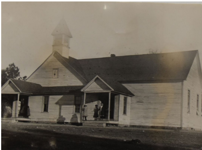
While the earliest extant institutional buildings were constructed of stone, the demolished Valdese Public School (1906-1922) is an example of an early frame institutional building. Photo courtesy of the Waldensian Heritage Museum Archives, Valdese, NC.
