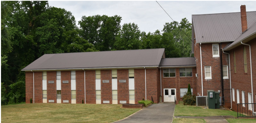
The ca. 1970s addition to the Mount Calvary Baptist Church (BK0659). Photo by author.
