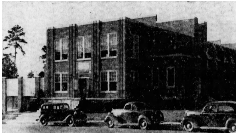
The original façade of the Francis Garrou Memorial Hall Community Center (BK0619). Photo from “Francis Garrou Memorial Hall,” The Charlotte Observer (Charlotte, North Carolina), October 27, 1943, Newspapers.com (accessed January 19, 2023).
