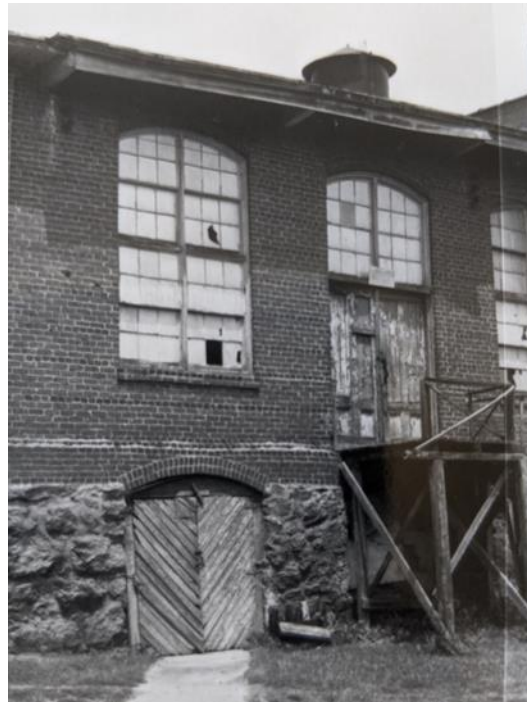
Figure 10. The Taylorsville Cotton Mill building featured a stone basement, arched window openings, and metal windows. Photo taken in 1984, in AX0050 Taylorsville Cotton Mill Survey File, HPO.
