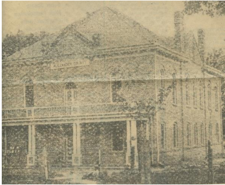
Figure 13. The 1902 Alexander County Courthouse. Photo ca. 1904. Courthouse Vertical File, Local History Room, Alexander County Library Main Branch.
