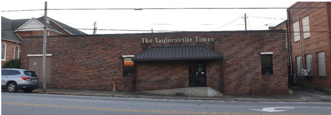
Figure 74. The Taylorsville Times building (AX0094). Top: Photo taken by Vickie Mason in 1986, AX0040 Survey File in HPO. Bottom: Photo by author.
