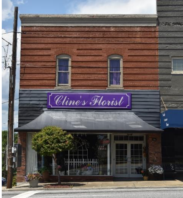
Figure 23. AX0099 features distinctive projecting brick bands. Photo by author.
