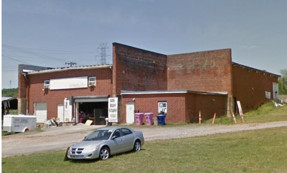
Figure 36. This utilitarian building may be all that remains of the Barnett Hosiery Mill. 2016 image from Google Street View.
