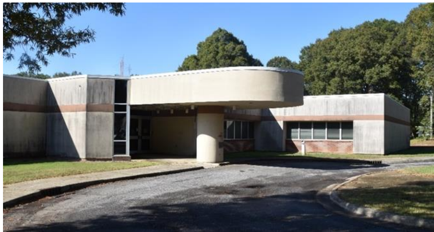
Figure 69. The ca. 1980 facade on the Alexander County Hospital. Photo by author.
