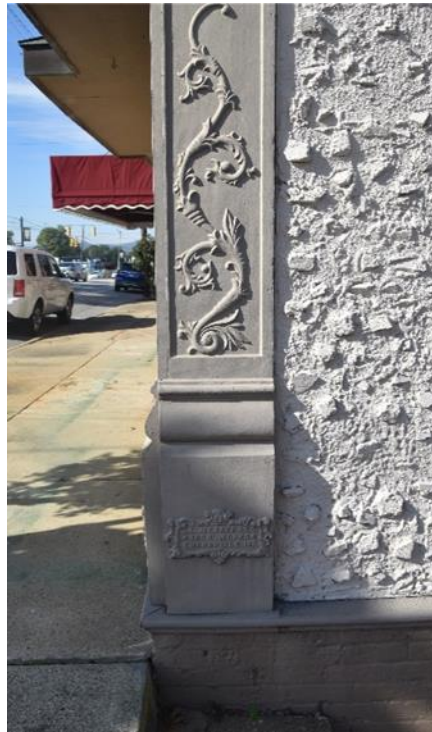
Figure 24. Cast iron column detail on People's Drug Store (AX0053). Photo by author.
