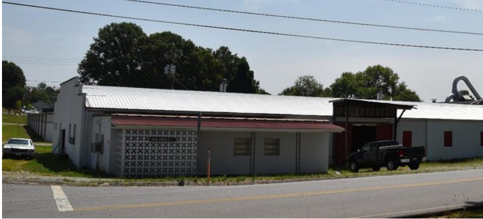
Figure 62. The Ideal Frame Company (AX0164) addition constructed ca. 1960. Photo by author.
