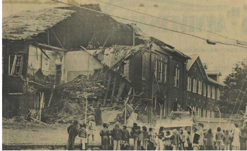
Figure 60. The former United Baptist Institute was demolished in 1976. United Baptist Institute & Taylorsville High School Vertical File, Local History Room, Alexander County Library Main Branch.
