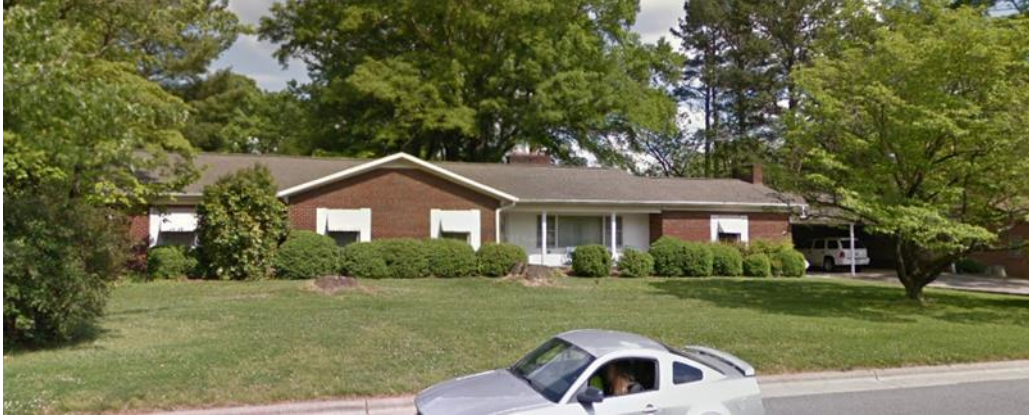
Figure 57. AX0168 is an early example of a typical Ranch house, a form that would become prolific in Taylorsville. The house has received an exterior renovation that has significantly altered its appearance since this image was created. Image from 2018 Google Street View.
