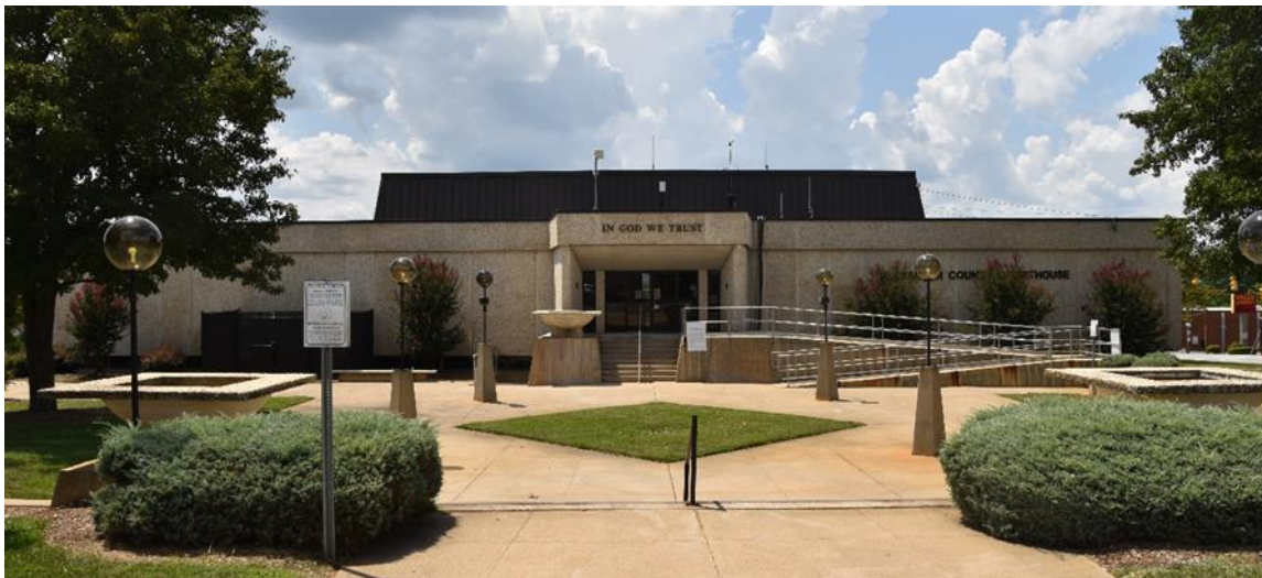
Figure 63. Alexander County Courthouse (AX0041) in 1976. Photo Boxes, Local History Room, Alexander County Library Main Branch.
