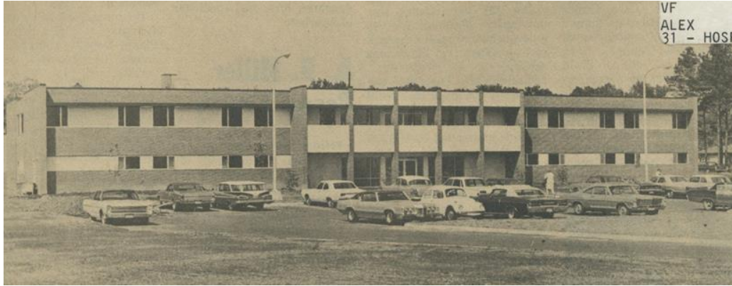
Figure 68. The Alexander County Hospital addition in 1973. Hospital Vertical File, Local History Room, Alexander County Library Main Branch.
