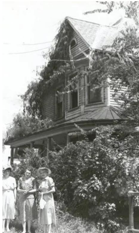
Figure 16. An undated photograph of AX0216 shows the original classical columns. Photo provided by Jeremiah Johnson.
