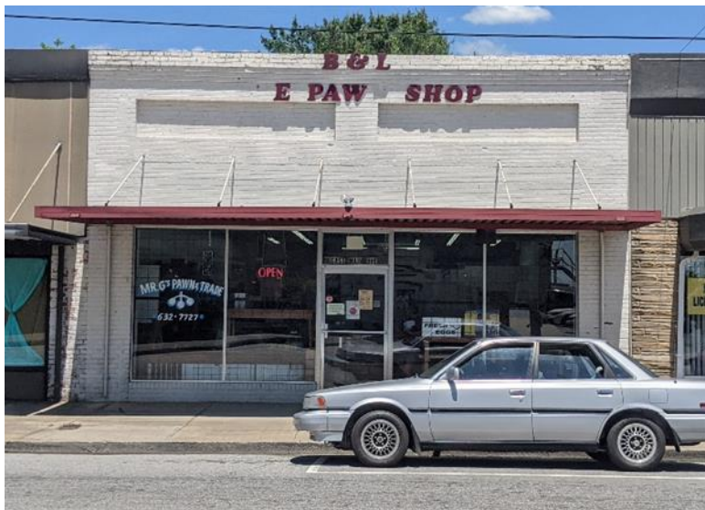
Figure 22. AX0115 features recessed brick panels, a detail common on downtown commercial buildings. Photo by author.
