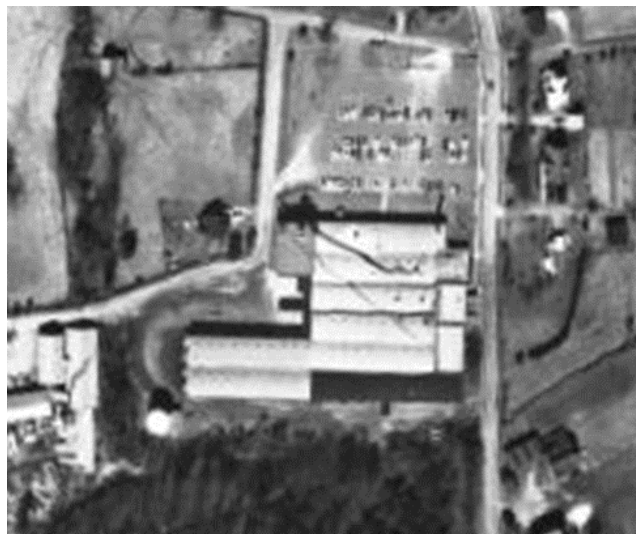
Figure 61. A 1972 aerial (right) shows the development of the Southern Paper Box Company (AX0171). The darker roof marks the early section with its bow-truss roof. Aerial photo from NCDOT Historical Aerial Imagery Index.
