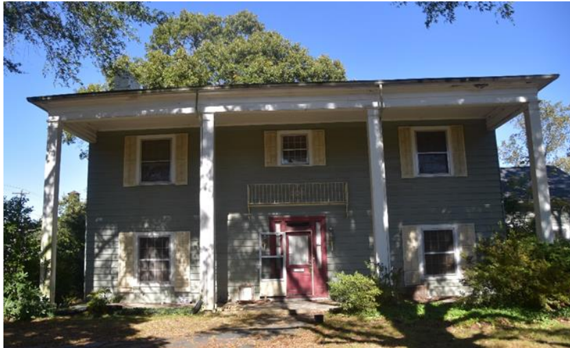
Figure 55. The Jennings House (AX0184) is a late example of a Colonial Revival-style house, evoking some of the earlier architecture of Taylorsville, such as the Thurston House (Figure 4). Photo by author.
