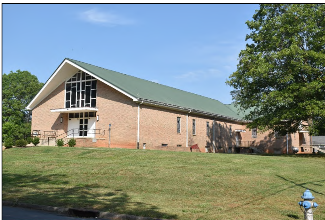
Figure 15. Trinity Presbyterian Church, 303 South Caldwell Street, facing west.
