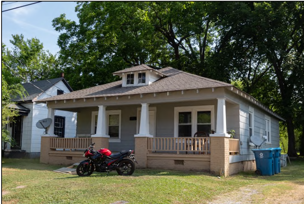
Figure 8. Example of a Craftsman-style residence, 616 West Marsh Street, facing northeast.
