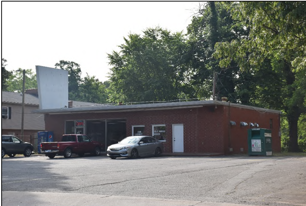
Figure 18. Laundromat, 813 South Fulton Street, facing east.
