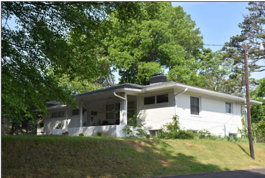
Figure 24. Example of building characterized as “1950-1975,” 324 South Caldwell Street, facing west.
