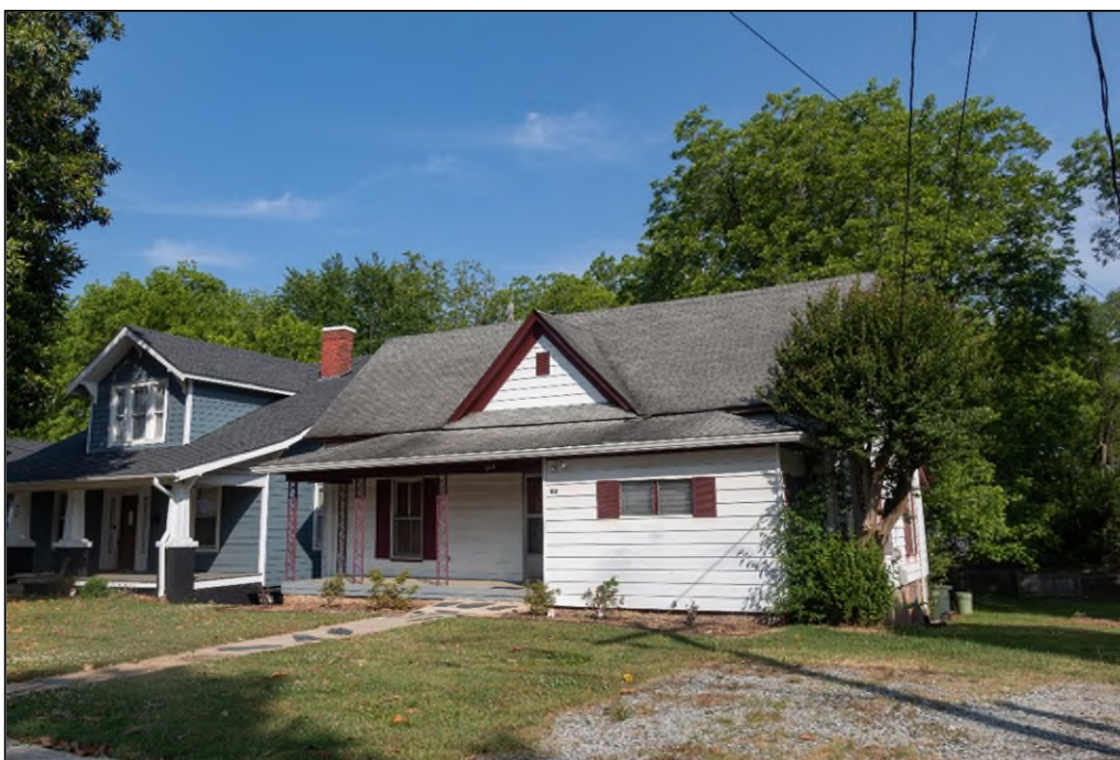
Figure 22. Example of building characterized as “Might Contribute,” 614 South Ellis Street, facing west.
