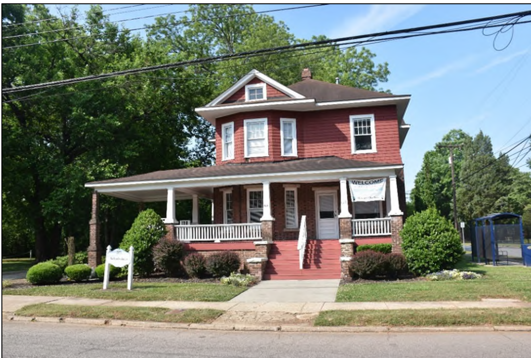
Figure 57. House at 629 West Monroe Street, facing southwest.
