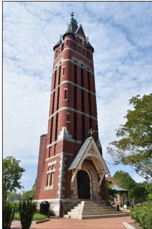
Figure 26. First Presbyterian Church Tower (RW1063), facing southwest.
