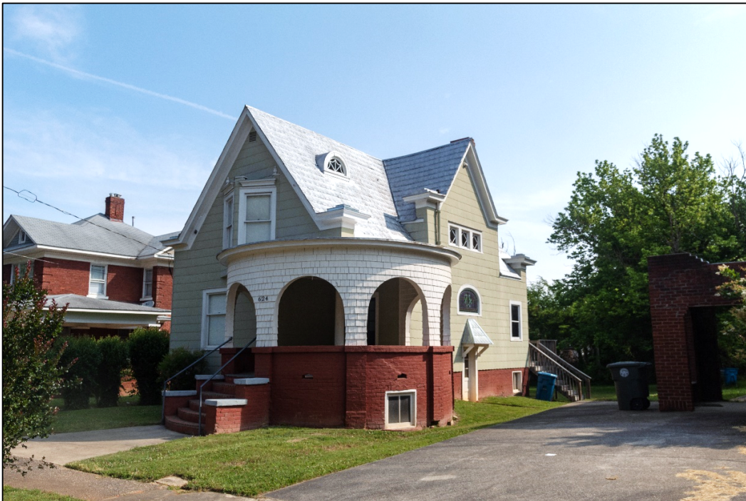
Figure 55. Mary A. Lynch House (RW0997), facing northwest.
