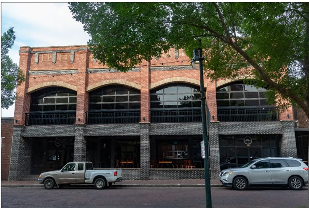
Figure 59. Mowery Building (RW2390), facing southwest.
