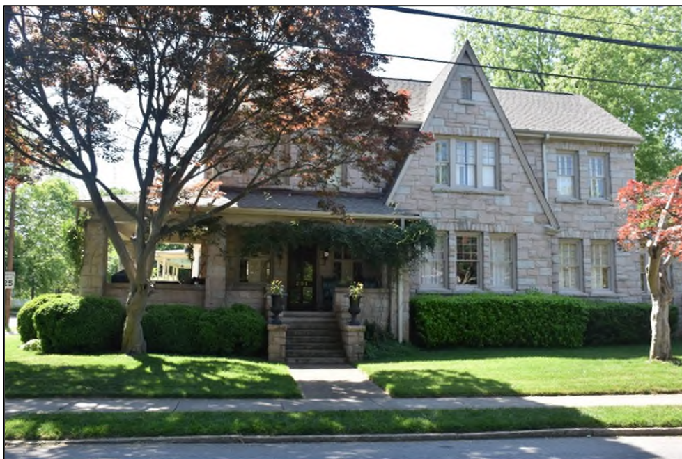
Figure 27. Hunt House (RW2277), facing south.
