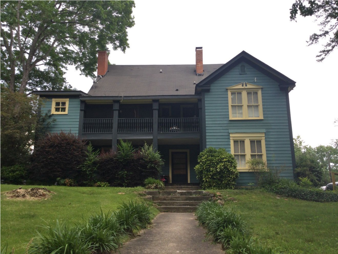
Figure 10. PL0220, Mooar Apartments, Tryon, constructed ca. 1890 as a boarding house.
