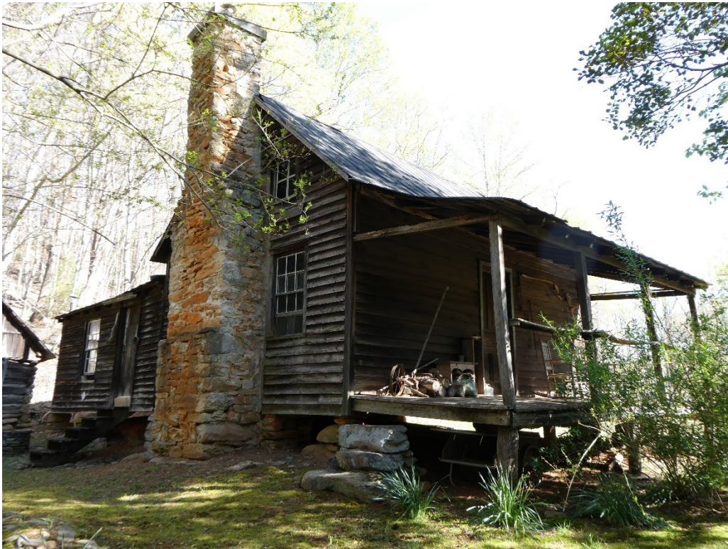
Figure 7. PL0011, John Hiram Johnson House, Saluda vic., constructed ca. 1887.
