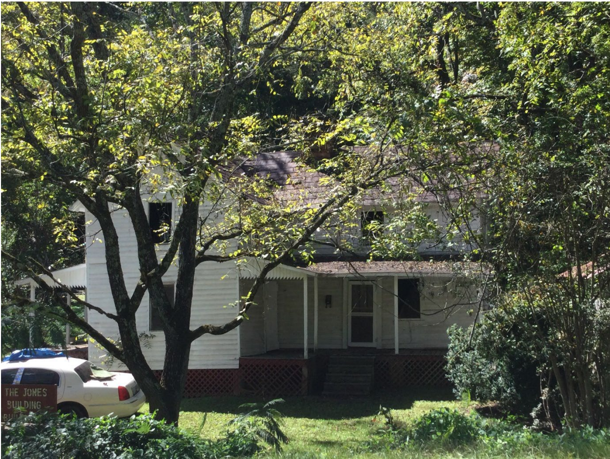
Figure 3. PL0010, Reverend Joshua D. Jones House, Stony Knoll/Mill Spring, constructed ca. 1897.
