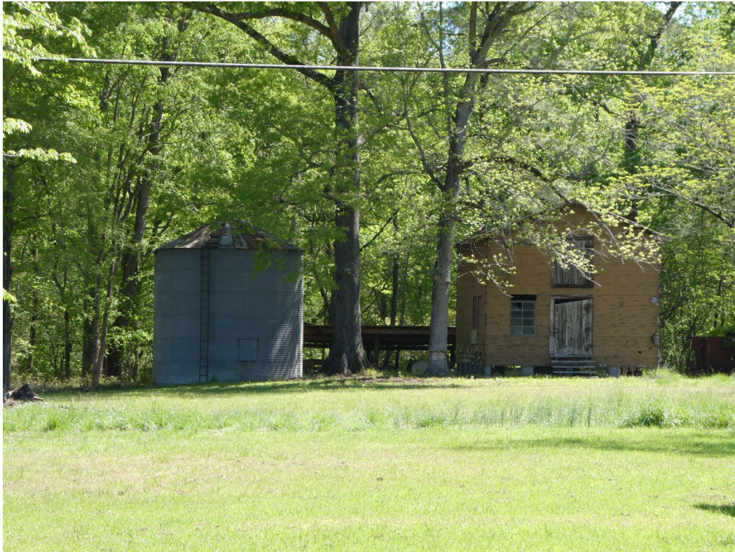
Figure 6: Grain Bin and Tobacco Packhouse at Averitt House property, CD1490. Photo by JMT.
