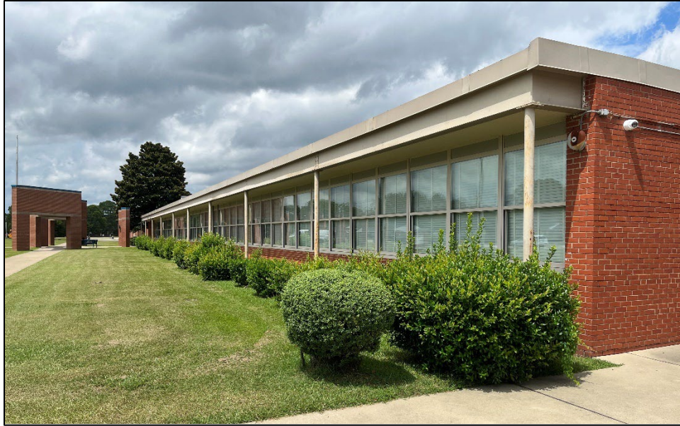
Figure 47. Ribbon windows on E. E. Smith High School (CD1520). Photograph by KDG, 2023.
