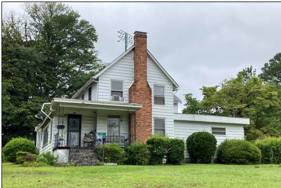
Figure 7. 1813 Broadell Drive. Photograph by KDG, 2023.
