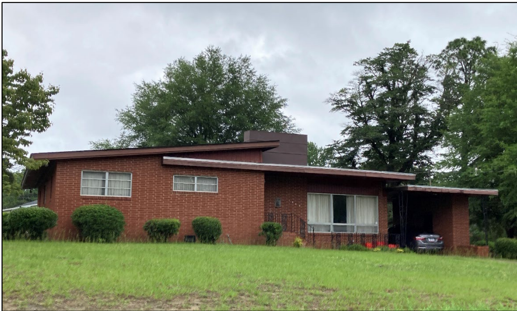
Figure 31. 1862 Broadell Drive. Photograph by KDG, 2023.
