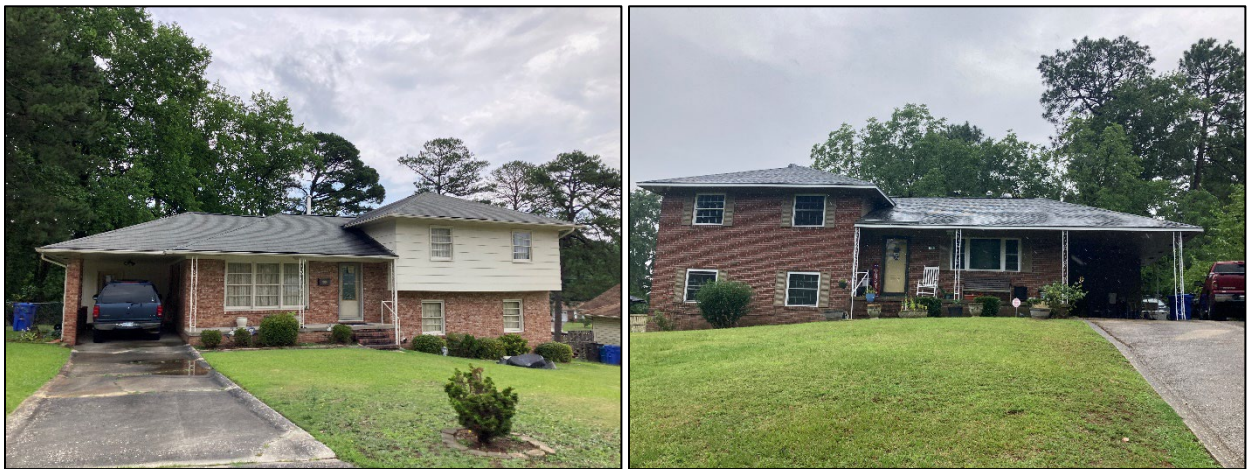
Figure 45. 1706 Eldridge Street (left) and 1822 Cascade Street (right). Photographs by KDG, 2023.
