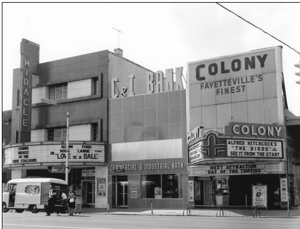
Figure 23. The Miracle and Colony Theaters on Hay Street in 1963. "From The Archives: A Century Of Downtown Fayetteville, 1900-2000," Fayetteville Observer , staff photo.
