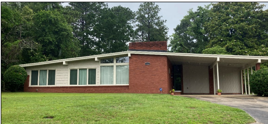
Figure 32. 526 Marion Court (CD1518). Photograph by KDG, 2023.
