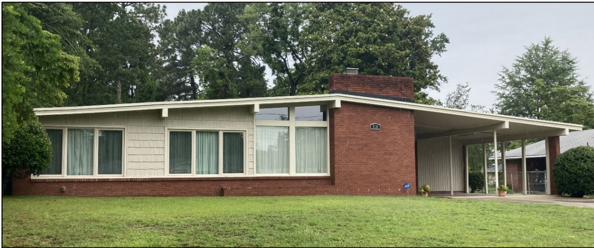
Figure 35. 526 Marion Court (CD1518). Photograph by KDG, 2023.
