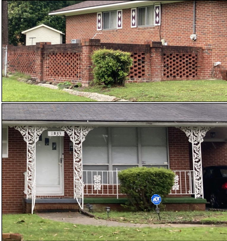
Figure 29. Examples of pierced brick walls and foliate wrought-iron columns. Top, 1855 Cascade Street, bottom, 1833 Gola Drive. Photograph by KDG, 2023.
