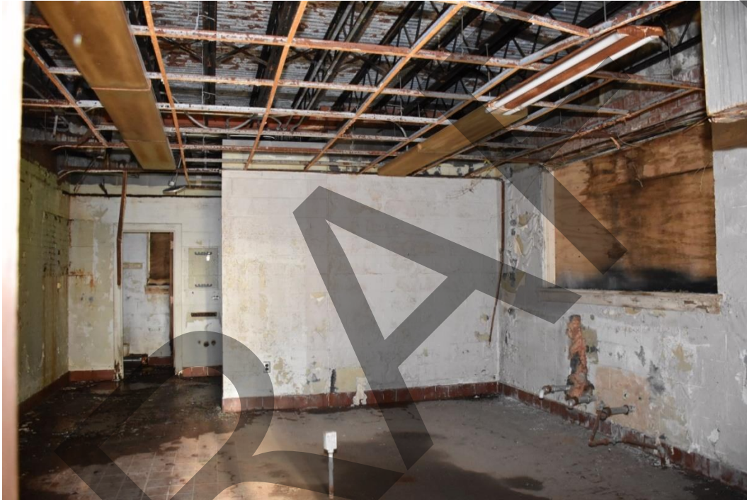
8. Kitchen in 1969 addition, looking east
