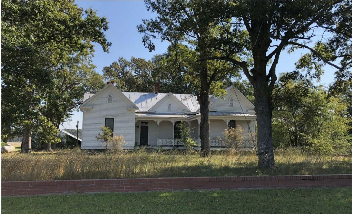
Façade, View to East.
