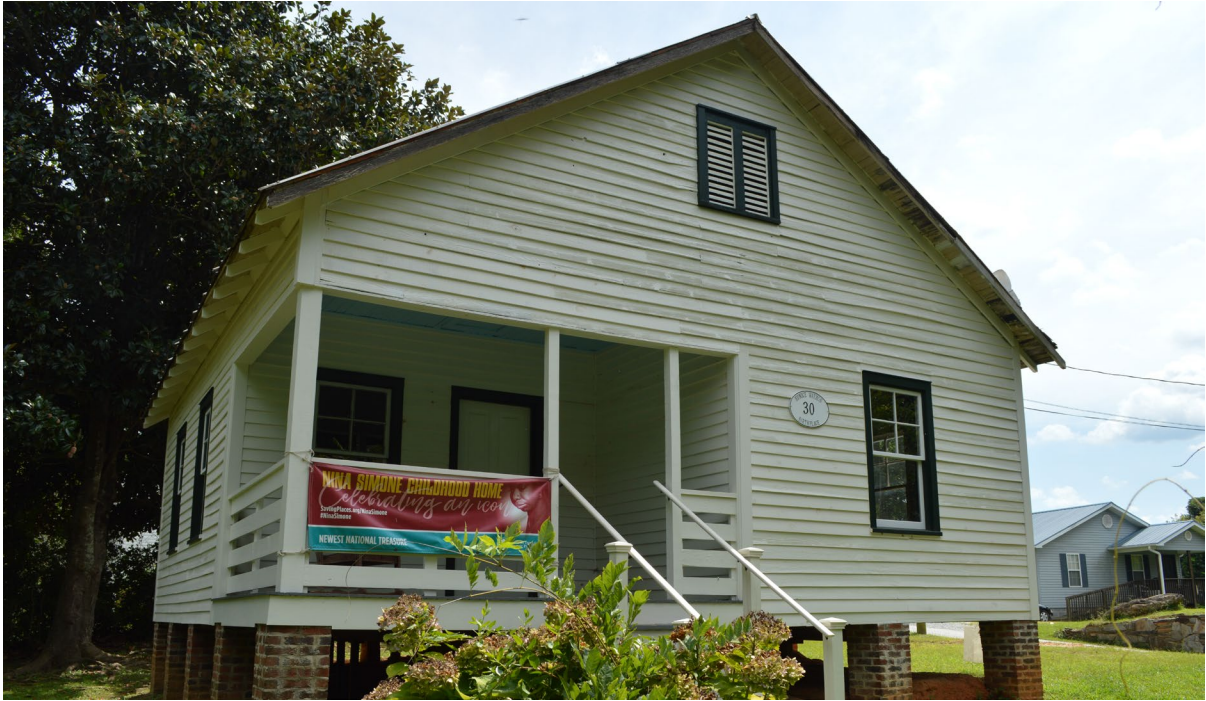
Eunice Waymon Birthplace, 30 E. Livingston Street, Tryon, NC. Oblique view of North corner, front (northwest) and northeast side elevation looking south.
