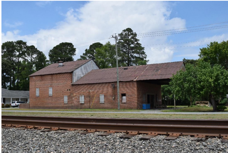
Overall view of front (south) elevation, looking NW.
