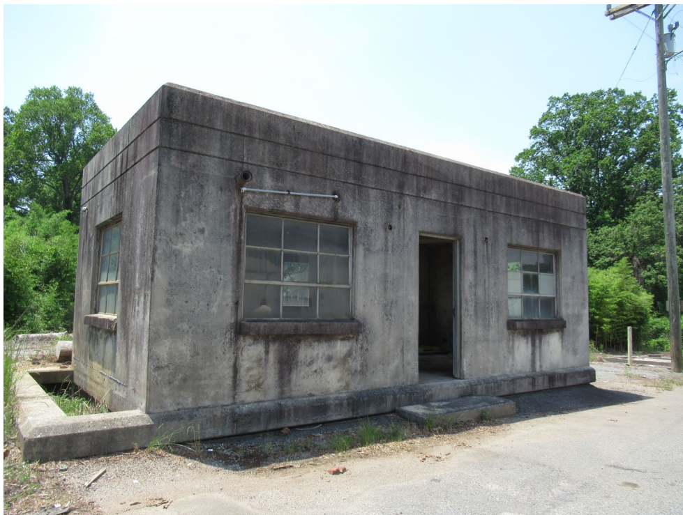
Chemical Feed House, View to SW
