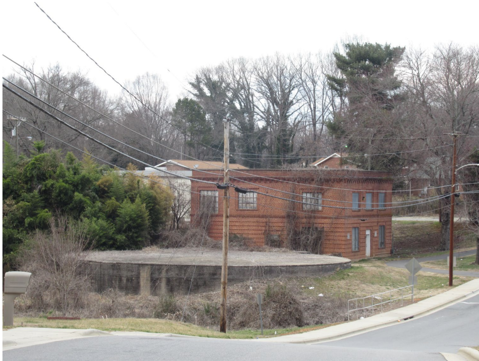
Pump House & Reservoir, View to NW
