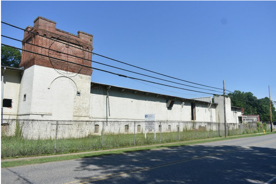
Façade, north end of the mill, view to northwest.
