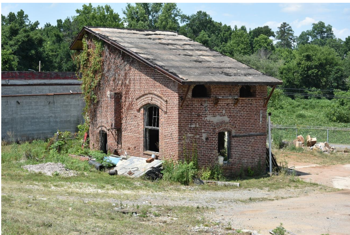
Transformer house, oblique rear view to northeast.
