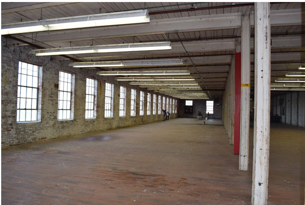
1935 addition, 3 rd floor, view west
