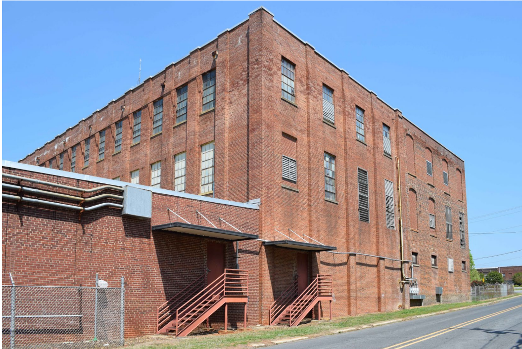
Oblique view showing 1953 addition, 1935 addition, and 1907 original building, view north
