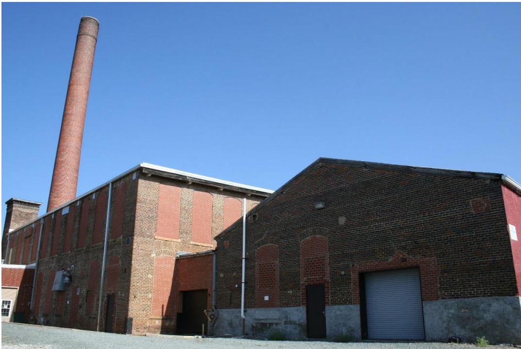
Dye House (Resource F), Picker House (Resource D), and Smokestack (Resource I) Facing north.
