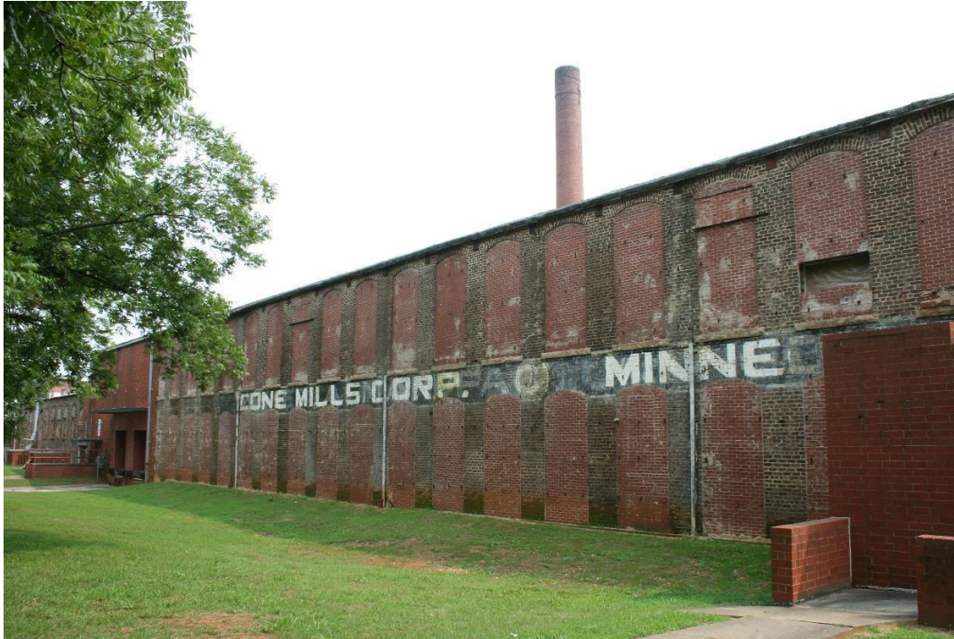
Mill #2 (Resource B) Facing southeast.
