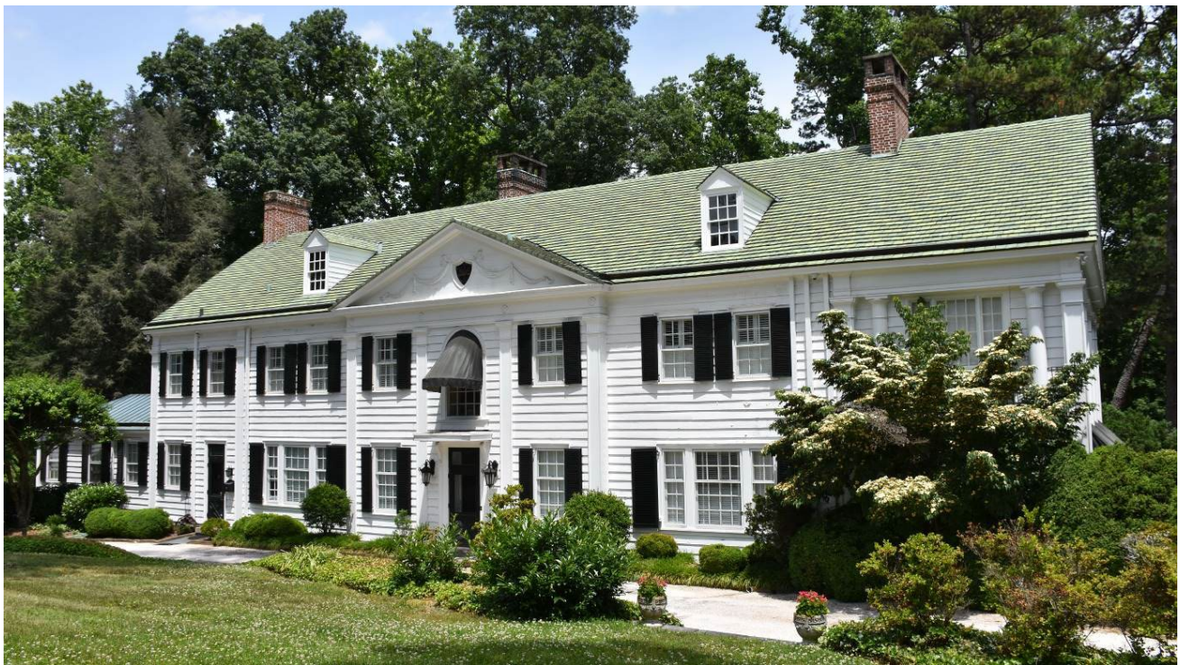
1. Façade (west elevation)
