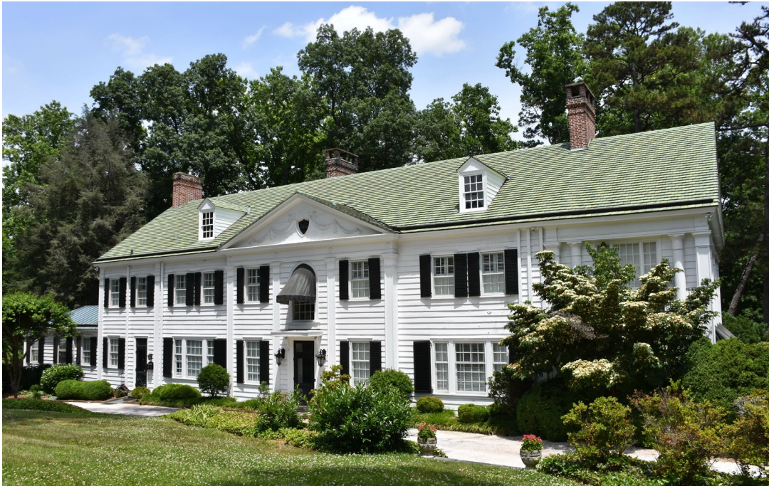
Façade (west elevation)
