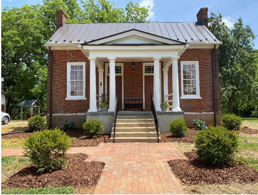
Front (north) elevation of structure showing restored columns, double entrances.
