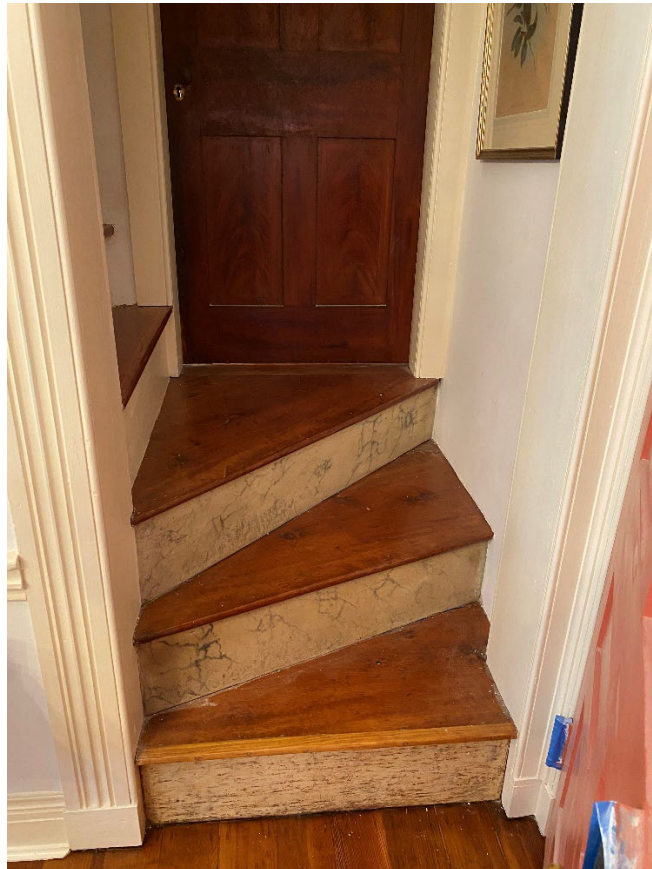
View of faux marbling on the stair risers in the west parlor staircase.
