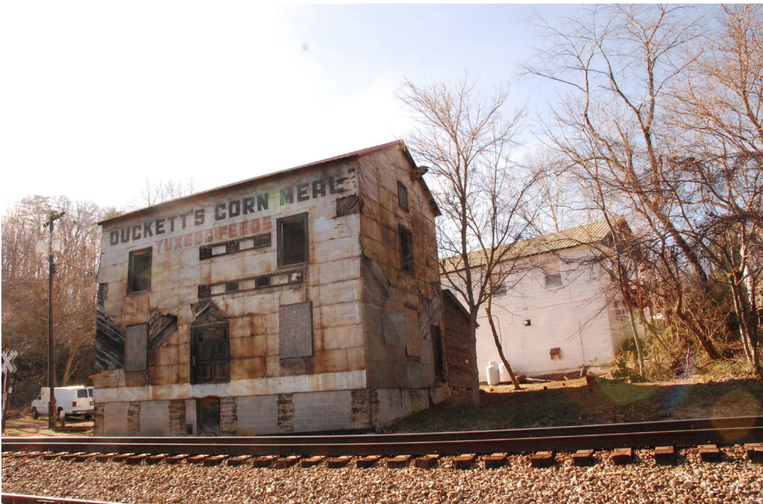
Craggy Historic District – View west across tracks toward Craggy Milling Company (l) prior to application of Tyvek house wrap and Red Men's Hall (r)
