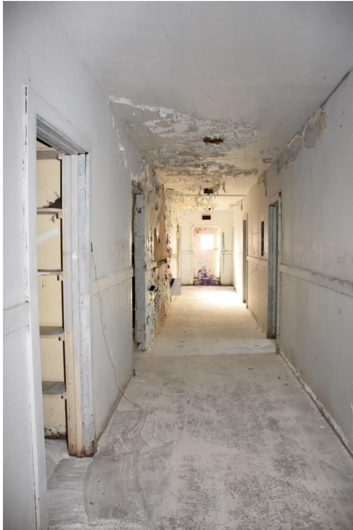
9. Second floor corridor, looking west
