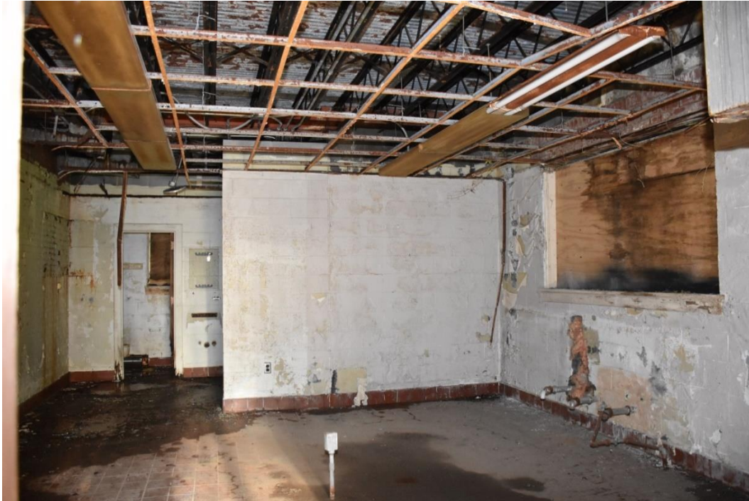
8. Kitchen in 1969 addition, looking east
