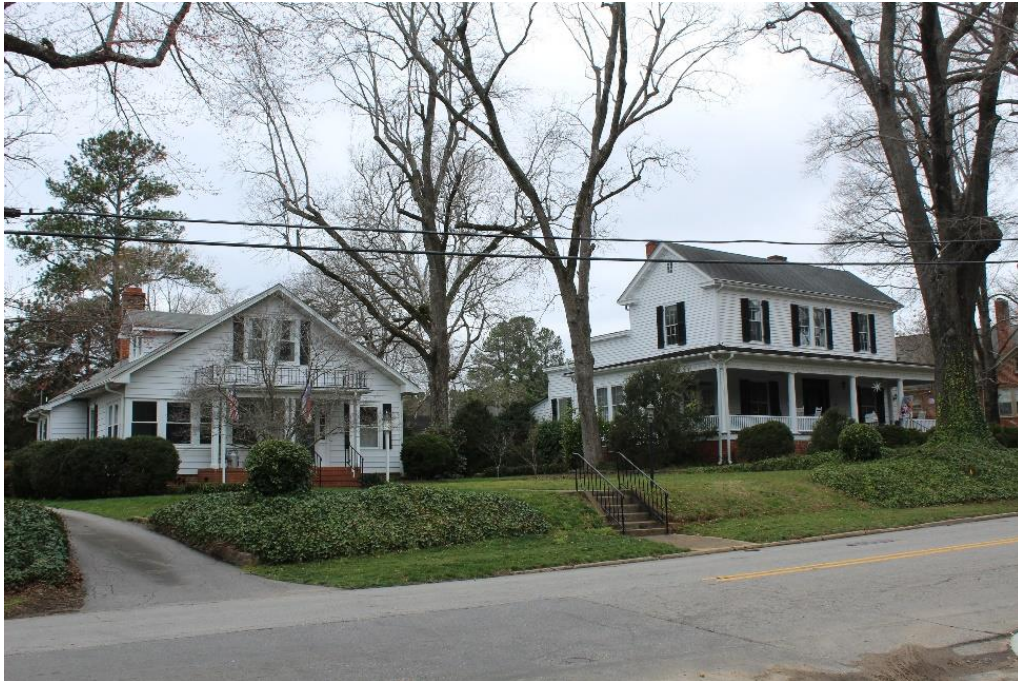
315-319 South Main Street, Warrenton Historic District Additional Documentation, Facing northeast.
