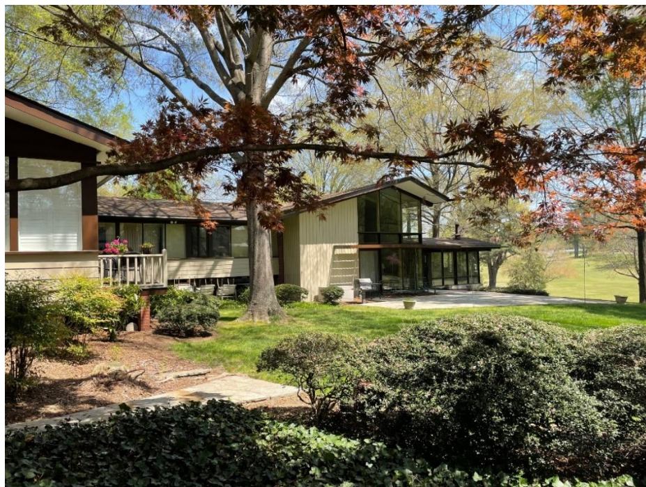
Photo #16 – South - West with 1955 & 1993 Additions
