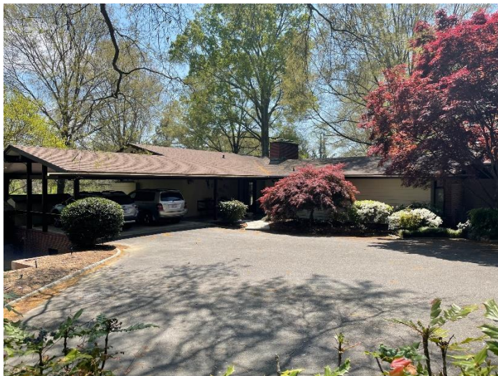
Photo #5 – Entrance Drive & Carport North Elevation
