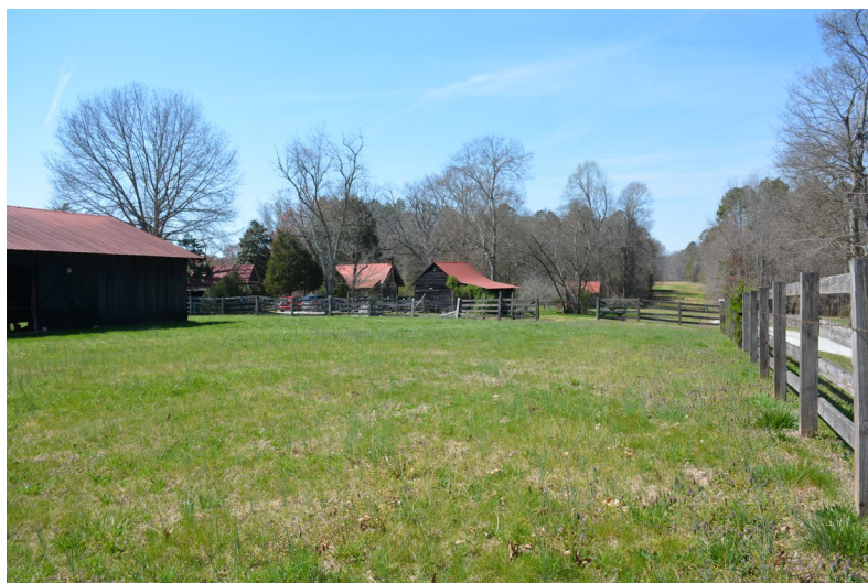
Group of outbuildings--barn, corncrib, cabin, and workshop--at northeast rear of property, view to west.
