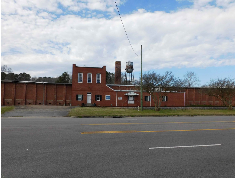
Main Building (Factory), Façade/Southeast Elevation, two-story c.1908 and one-story c.1989 Office in foreground, Camera facing Northwest
