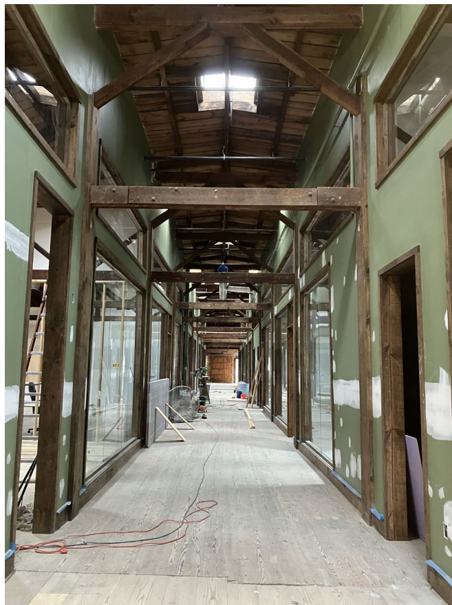
Interior, Central Corridor, View to South
