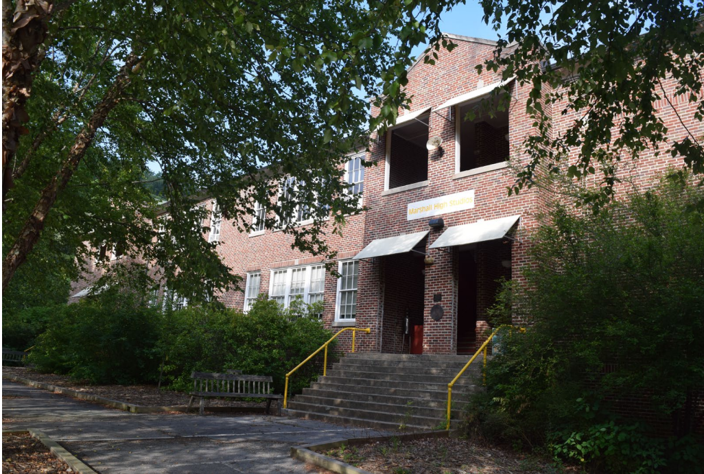
High School, east elevation/entry, view southwest.
