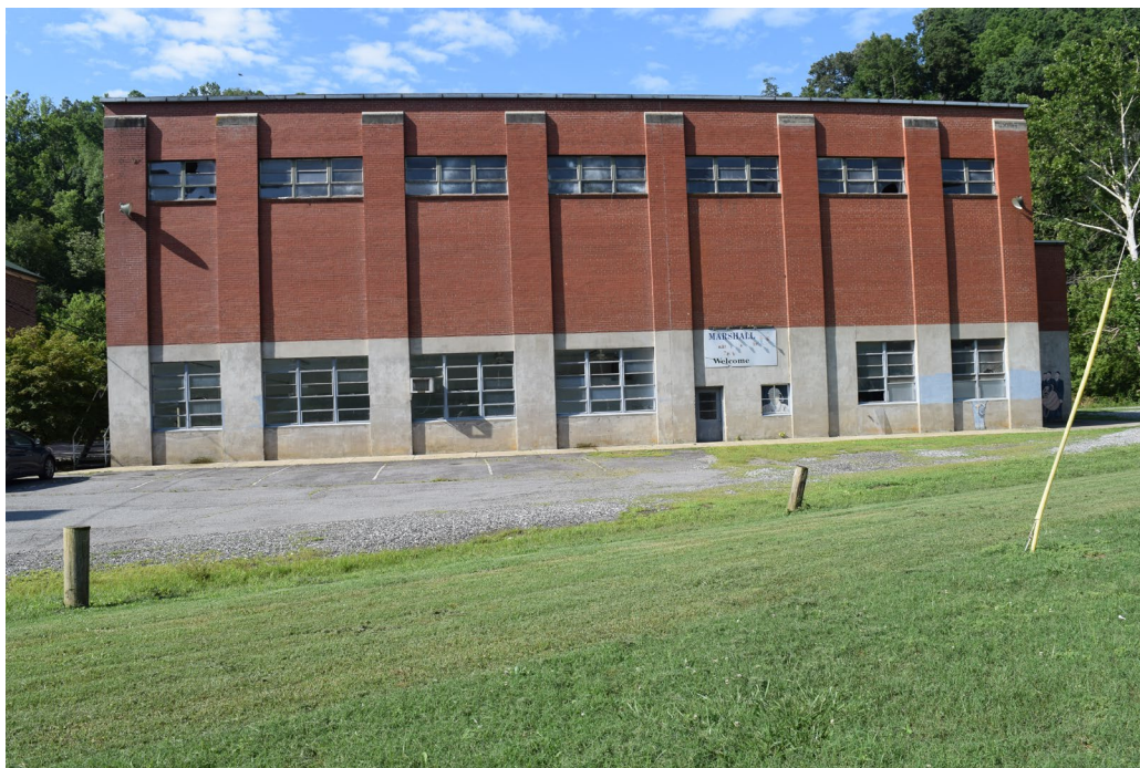
Gymnasium, north elevation, view south.
