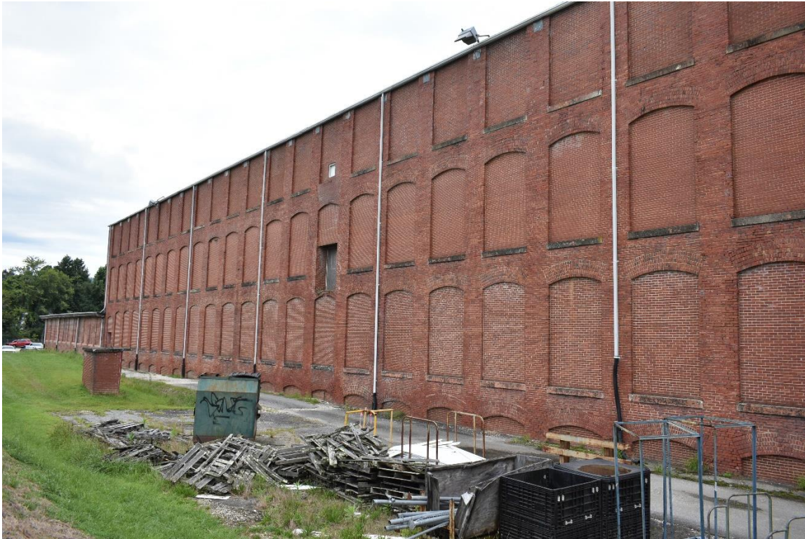
Mill No 2, east side elevation, view to southwest.
