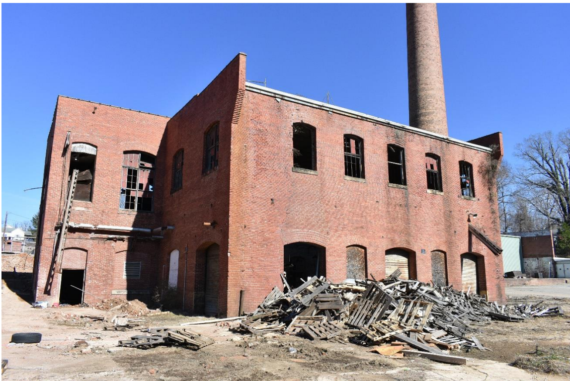
Boiler House, oblique view to northwest.
