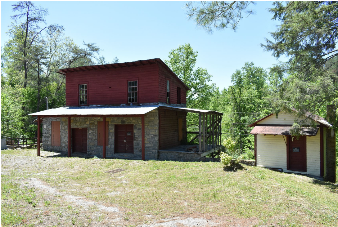
Stepp's Mill and Saconon Post Office, facades, view to southwest
