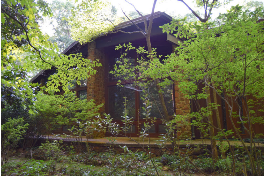
Façade, view north.
