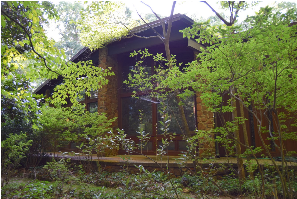
Façade, view north.
