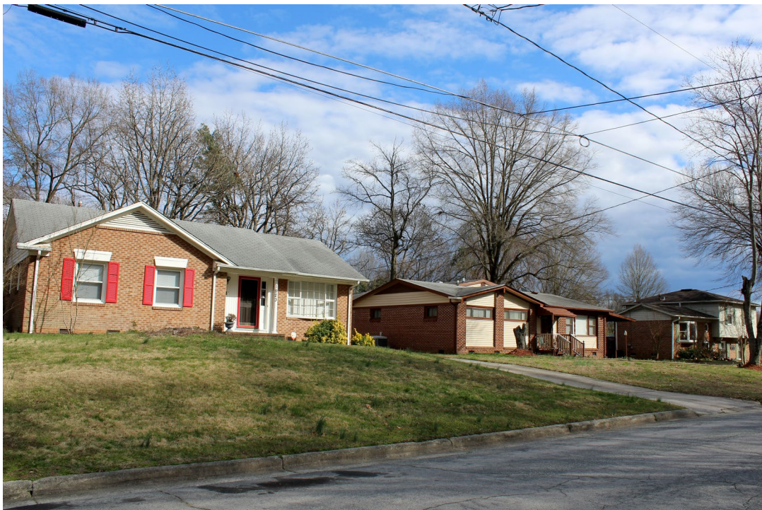
1923-1927 Carlton Avenue Facing southeast
