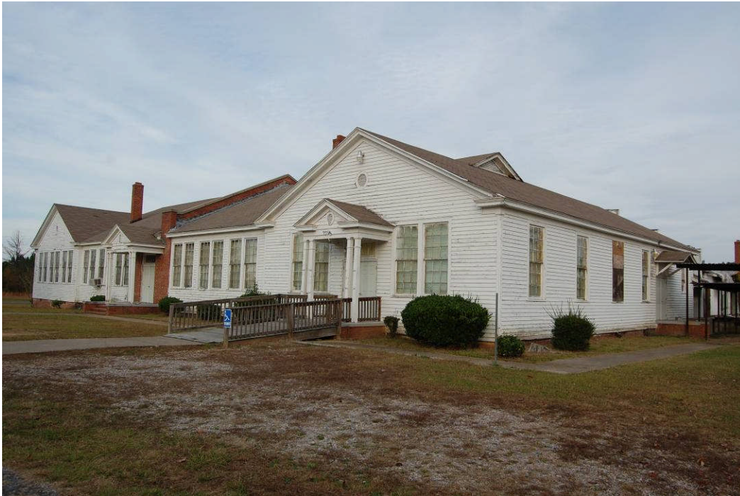
Overall view of 1941 school building
