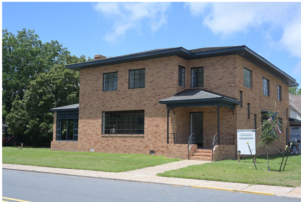
East and north sides of house, view facing west.
