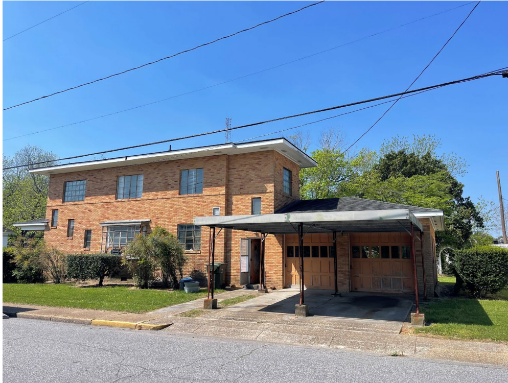
South (front) and east sides of house, view facing northwest.
