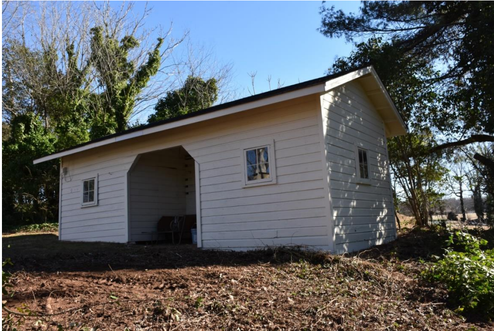
17. Stable, northwest oblique
