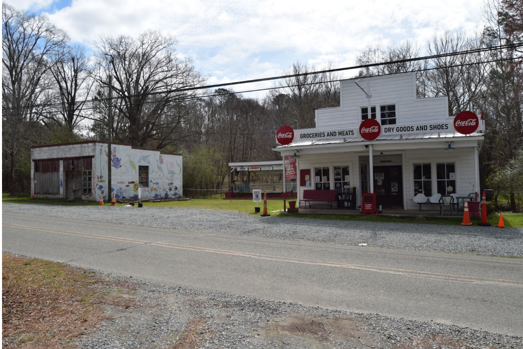
View S toward J.G. Williams Store (R) with Auto Repair Garage (L).
