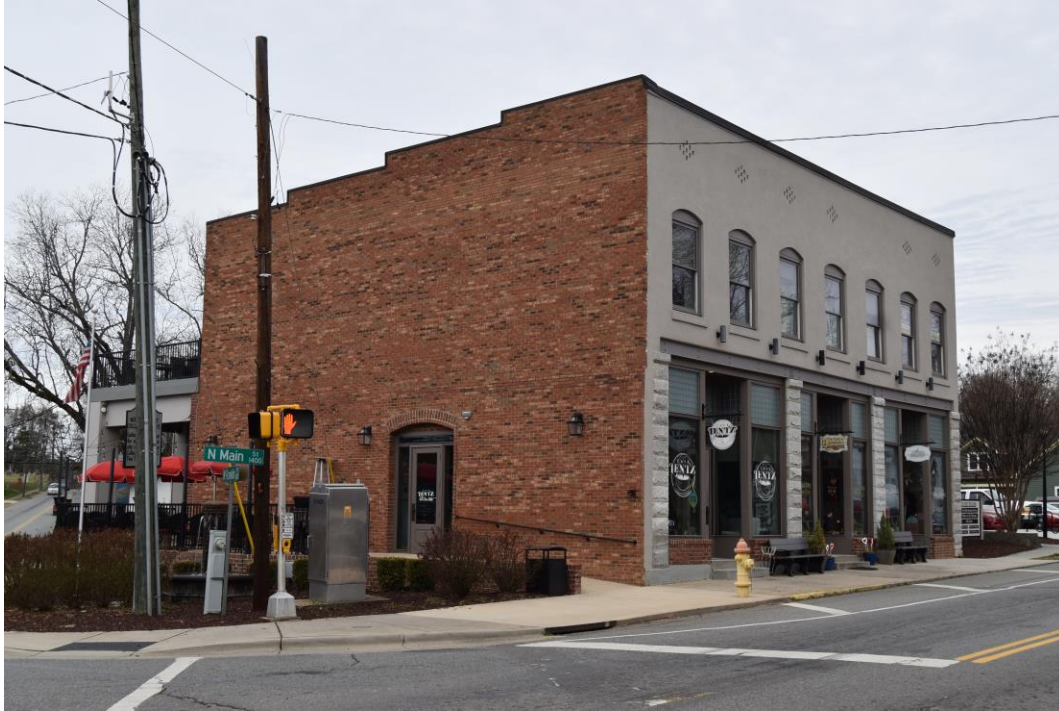
Mount Pleasant Town Hall/Commercial Building, 1448-1462 North Main Street facing northwest
