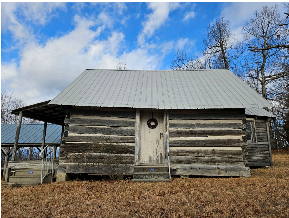
Walker Top Baptist Church, south-southeast elevation, camera facing north-northwest
