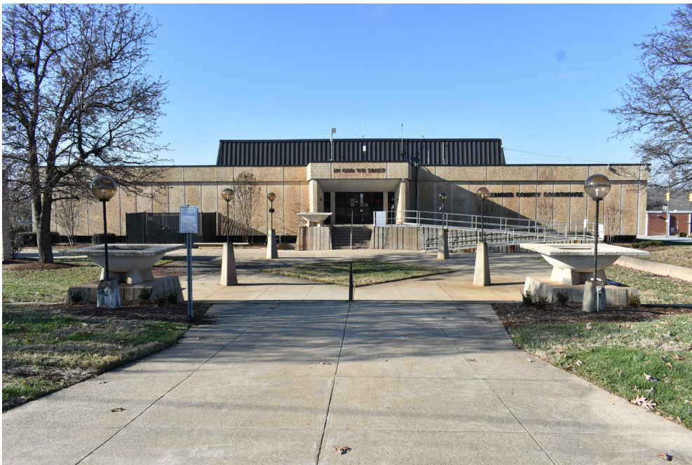
Alexander County Courthouse, 27 West Main Avenue, view to west
