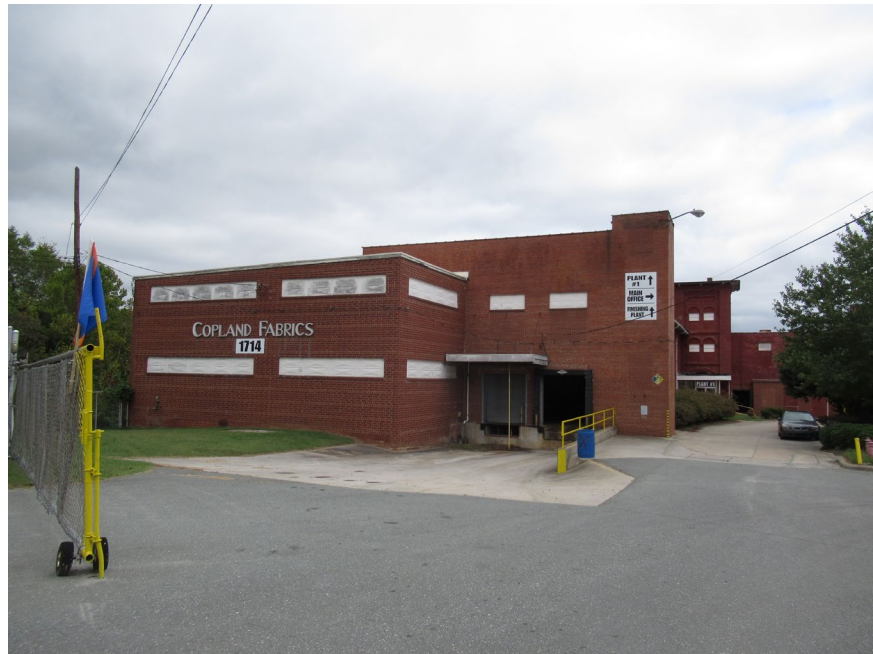
Exterior of Main Mill, West Elevation, View to East
