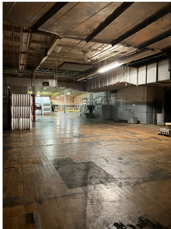
Interior, Mill Two, Main Level, View to Northwest
