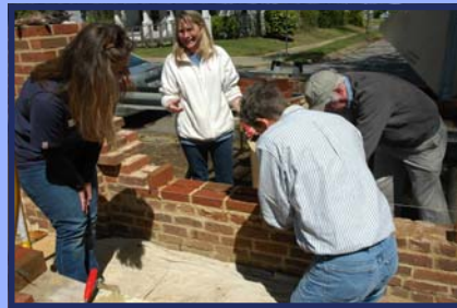
Brick Restoration Workshop Raleigh National Cemetery
