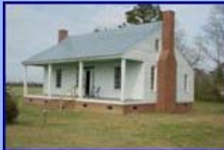
William Phillips House Currently undergoing restoration
