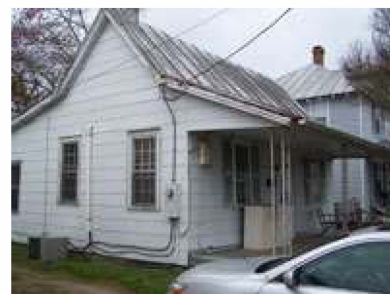
304 East Queen Street, Edenton, before rehabilitation work began
