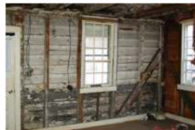
Early interior finishes
