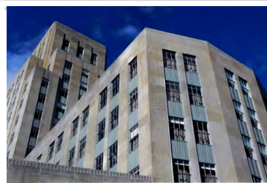
The Hill Building Durham / Durham Co.
