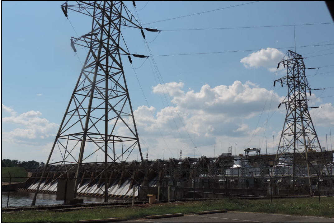
Figure 4: Tillery Dam and Hydroelectric Plant (MG0029, DOE 2006), Lake Tillery
