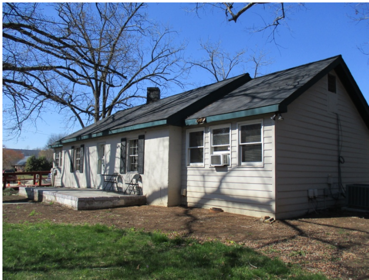
WA7936 House, 10200 Durant Road
