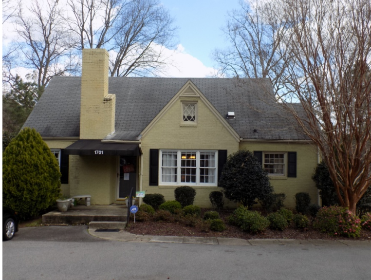
WA937 House, 1701 Jones Franklin Road
