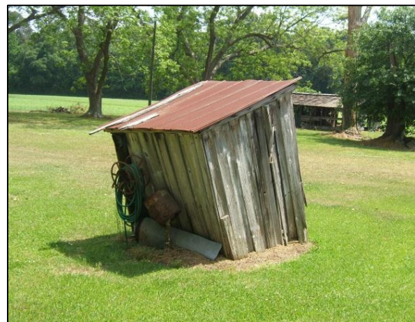
Figure 33 – Pump house at 130 Garden Road, PD0321
