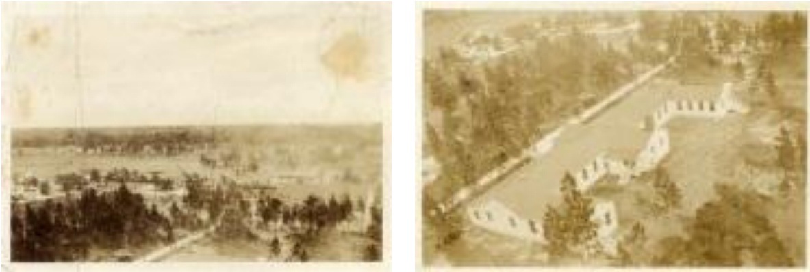
Figure 12 - Views from the watertower showing progress at the Penderlea community center including the school buildings on the left and the cafeteria on the right. (Photo provided by Ann Cottle)
