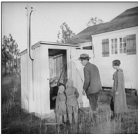
Figure 32 – Pump house in 1936 (Library of Congress)
