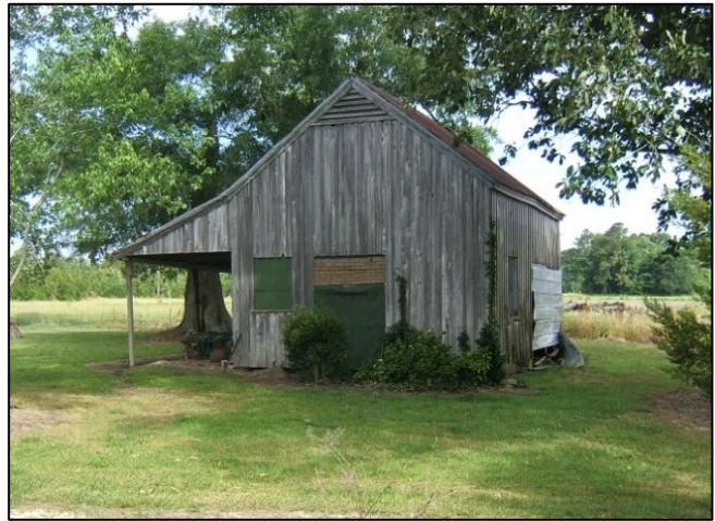
Figure 36 – Original Penderlea barn at 5135 Penderlea Highway, PD0351
