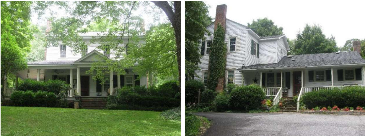
Figure 1: Front façade (left) and side façade (right) of the Elias R. Powell House (CW0393) at 807 Lower Creek Drive
