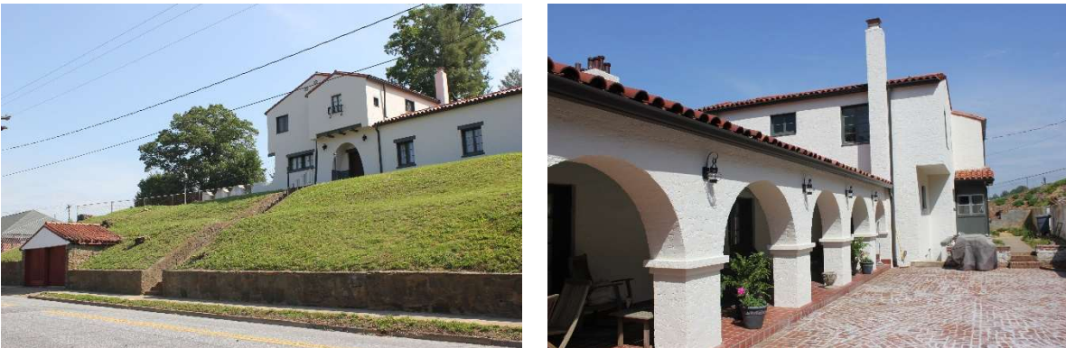
Figure 40: Two views of the Galvin-Templeman House (CW0676) at 211 Mulberry Street
