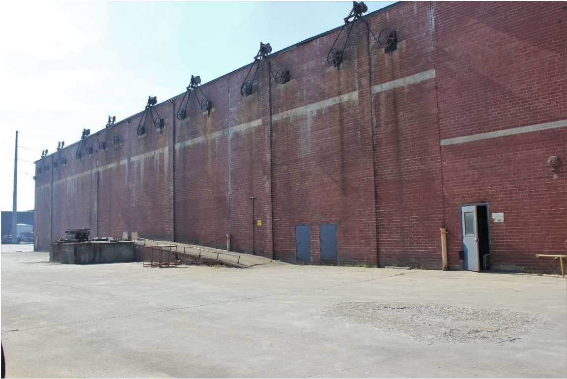
Figure 49: Former drying kilns at Bernhardt Plant #5 (CW0825) at 1904 Morganton Boulevard
