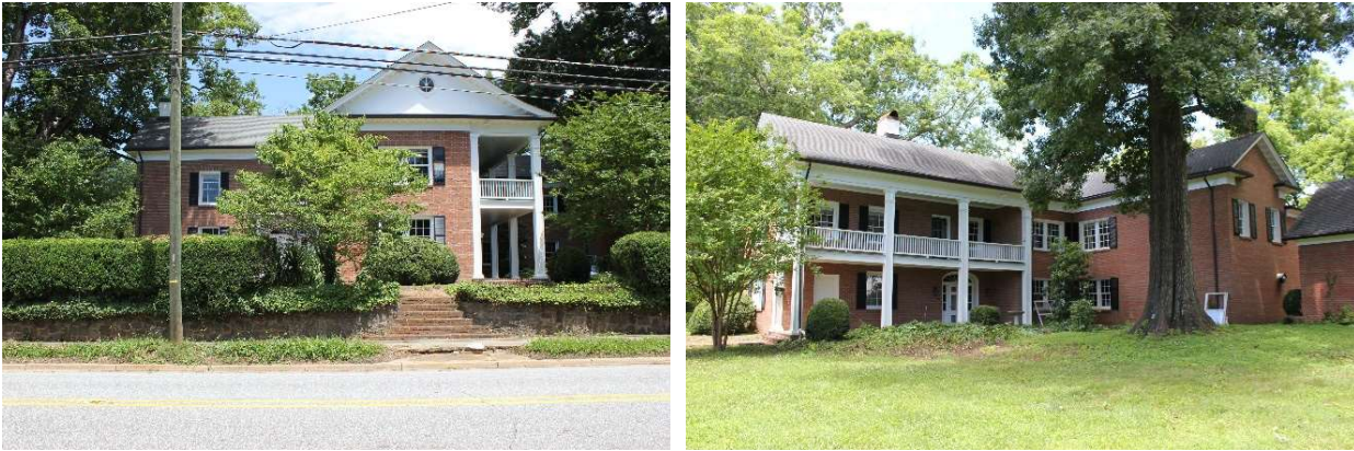
Figure 3: Front façade (left) and side façade (right) of the James Harper House (CW0383) at 1436 West Harper Avenue
