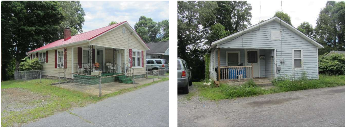
Figure 29: 517 Hartley Place (CW0597) on left and 519 Hartley Place (CW0598) on right
