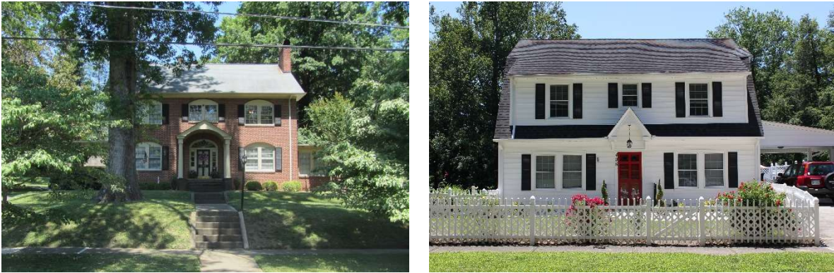
Figure 39: 407 Norwood Street (CW0640) on left and 406 Norwood Street (CW0639) on right
