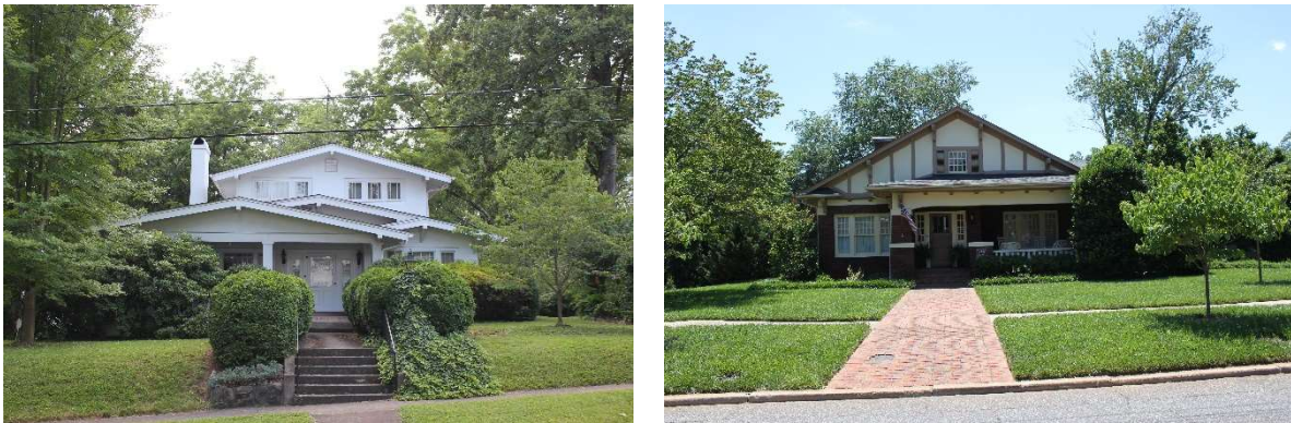
Figure 36: James C. Hogan House (CW0390) at 416 Hibriten Avenue on left and the Garland Jones House (CW0396) at 430 Norwood Street on right
