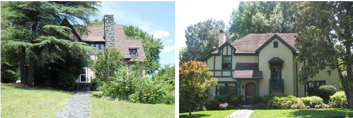
Figure 46: 515 Mulberry Street (CW0679) on left and the Edward Crisp House (CW0398) at 504 Norwood Street on right
