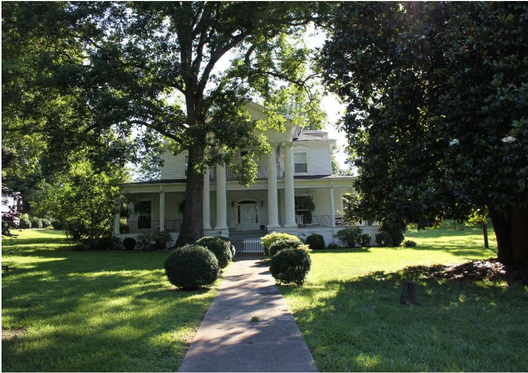
Figure 22: Mark and Mary Squires House (CW0395) at 221 Mulberry Street
