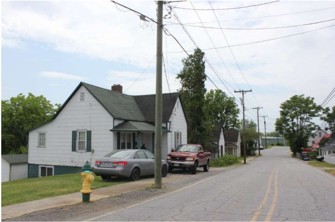
Figure 18: View of mill housing along Underdown Street
