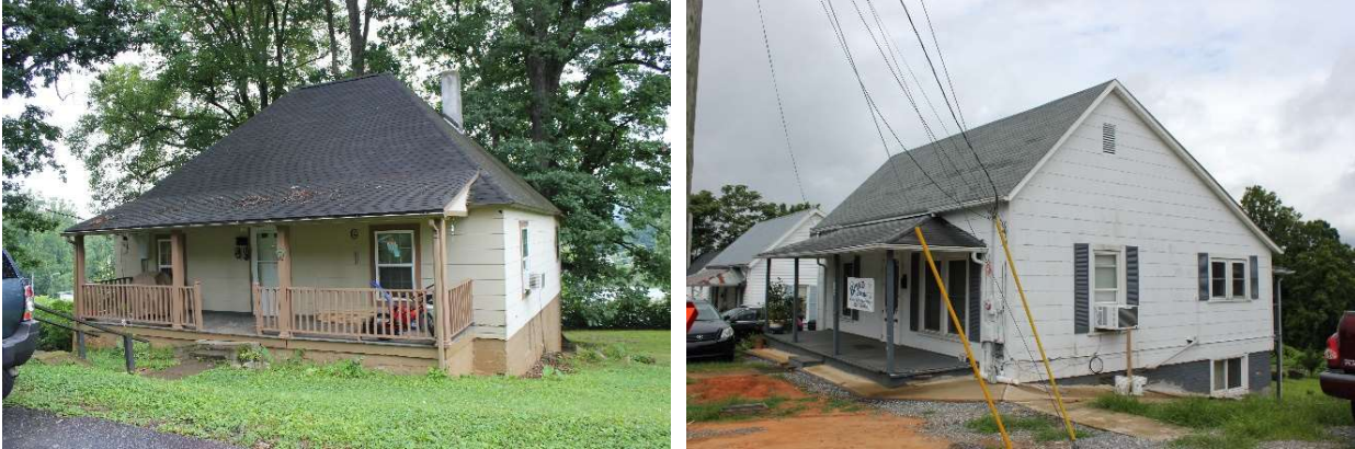
Figure 19: 1232 Spainhour Street (CW0819) on left and 1324 Underdown Avenue (CW0821) on right
