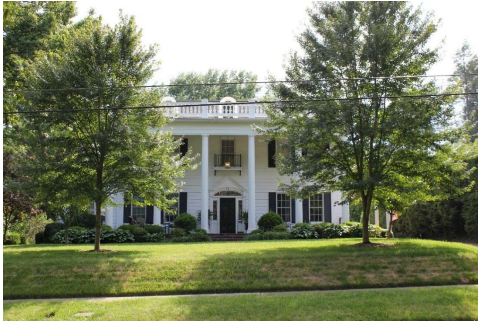
Figure 41: L. Spurgeon Spurling House (CW0696) at 414 Hibriten Avenue
