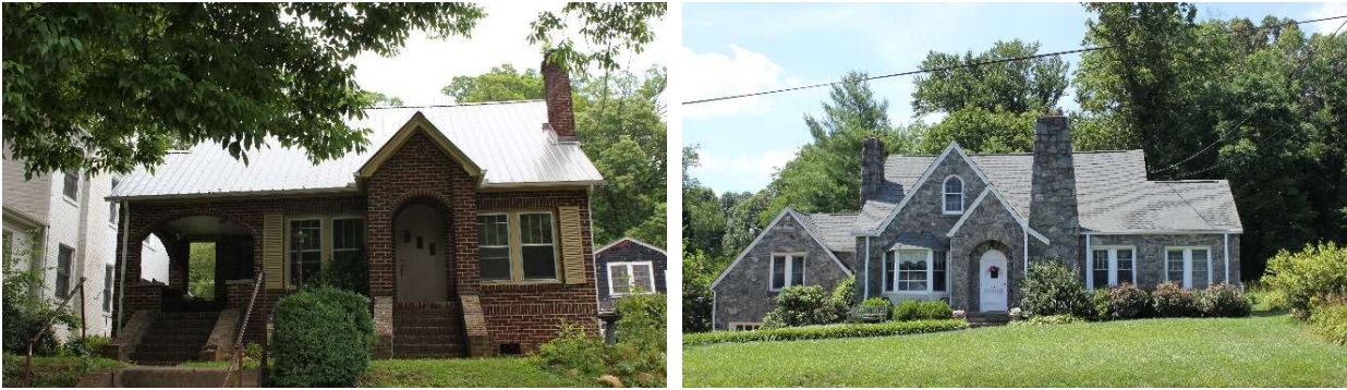
Figure 47: 215 Norwood (CW0621) on left and 628 Pennton Avenue (CW0736) on right
