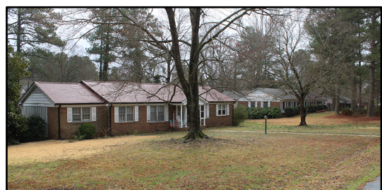
Figure 22: Cardinal Hills (WA4989) 200-block Mockingbird Lane
