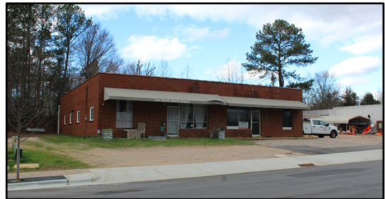
Figure 17: Commercial Building (WA8723) 502-504 South White Street
