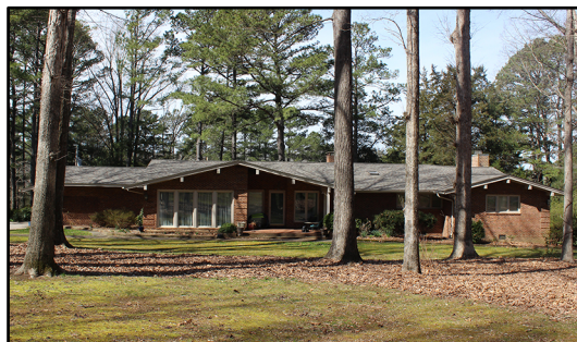
Figure 24: C. R. and Lillian Faircloth House (WA8695) 1414 Country Club Drive
