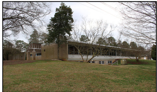
Figure 18: Northern Wake Hospital (WA8705) 250 South Allen Road
