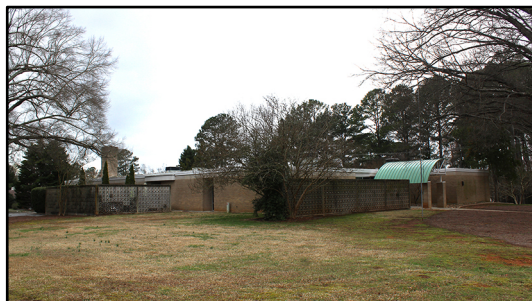
Figure 11: Northern Wake Hospital (WA8705) 250 South Allen Road
