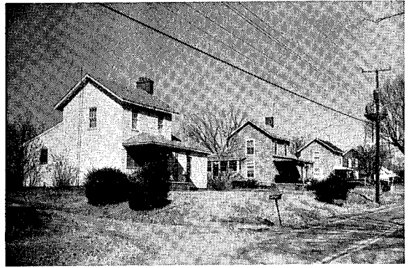
SITE NAME: Swepsonville Mill House LOCATION: Thompson AGE: c. 1880 BUILDING MATERIAL: Frame CHIMNEY: Brick
