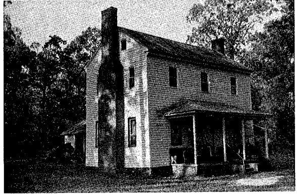
SITE NAME: R. E. Green House LOCATION: Coble AGE: c. 1830 FLOOR PLAN: 2 BUILDING MATERIAL: Frame CHIMNEY: Brick
