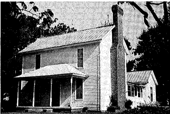
SITE NAME: Riley Shepherd House LOCATION: Coble AGE: c. 1880 FLOOR PLAN: 2 BUILDING MATERIAL: Frame CHIMNEY: Brick
