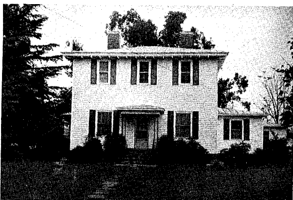
SITE NAME: Paisley-Cates House LOCATION: Melville AGE: c. 1815; Remodelled c. 1850 FLOOR PLAN: 2 BUILDING MATERIAL: Frame CHIMNEY: (?) Original Gone; Brick
