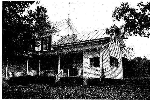
SITE NAME: Jacob Long Log House LOCATION: Graham AGE: (?) Reported 1761 FLOOR PLAN: 1 BUILDING MATERIAL: 1 CHIMNEY: Brick
