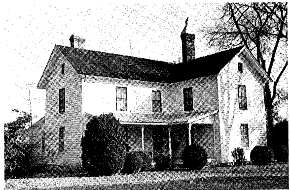
SITE NAME: Stanley Coble House LOCATION: Patterson AGE: c. 1858 (oldest part) FLOOR PLAN: 2A BUILDING MATERIAL: Frame CHIMNEY: Brick
