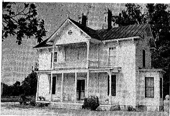
SITE NAME: Y. B. Warren House LOCATION: Faucette AGE: c. 1890 FLOOR PLAN: 6 BUILDING MATERIAL: Frame CHIMNEY: Brick
