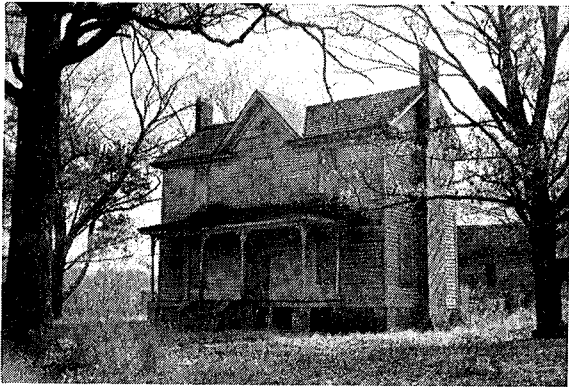
SITE NAME: William Tinin House LOCATION: Patterson AGE: c. 1885 FLOOR PLAN: 2 BUILDING MATERIAL: Frame CHIMNEY: Brick
