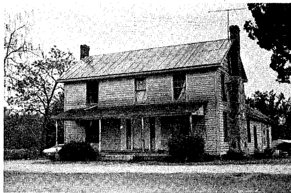
SITE NAME: Sol Martin House LOCATION: Pleasant Grove AGE: c. 1885 FLOOR PLAN: 6 BUILDING MATERIAL: Frame CHIMNEY: Stone, Brick
