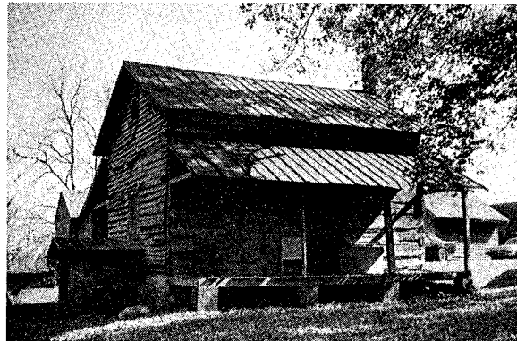
SITE NAME: Sharpe Nicholson Site LOCATION: Coble AGE: c. 1885 FLOOR PLAN: 2 BUILDING MATERIAL: Frame CHIMNEY: Brick
