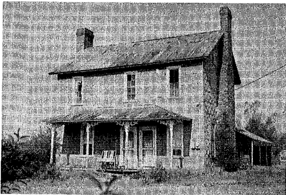
SITE NAME: S. A. Clapp House LOCATION: Patterson AGE: c. 1850 FLOOR PLAN: 2 BUILDING MATERIAL: Frame CHIMNEY: Brick
