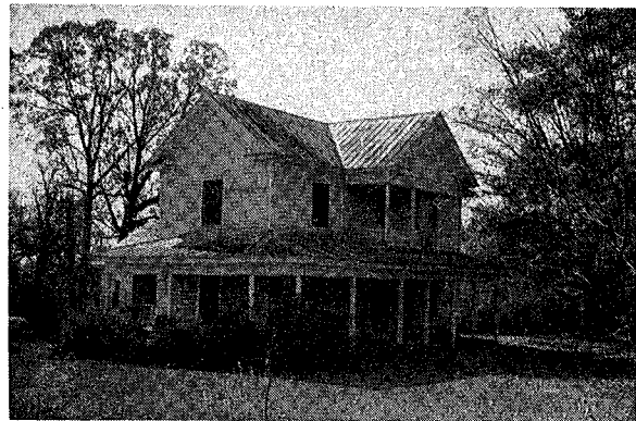
SITE NAME: A. McPherson House LOCATION: Patterson AGE: c. 1885 FLOOR PLAN: 6 BUILDING MATERIAL: Frame CHIMNEY: Brick
