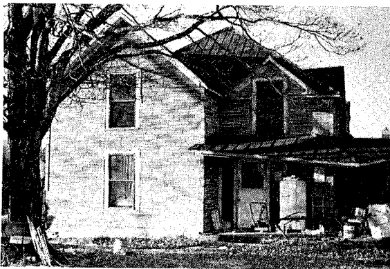
SITE NAME: Amick Foust House LOCATION: Albright AGE: (?) FLOOR PLAN: 1 (Original part) BUILDING MATERIAL: Log, Frame Addition CHIMNEY: Stone, Brick
