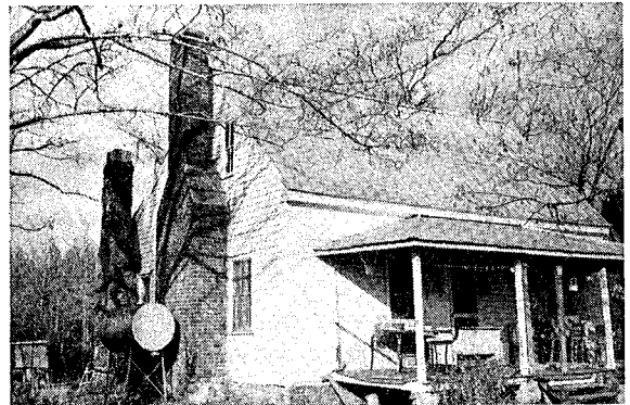
SITE NAME: Dixon-Thompson House LOCATION: Haw River AGE: c. 1860 FLOOR PLAN: 3 BUILDING MATERIAL: Frame CHIMNEY: Stone, Brick
