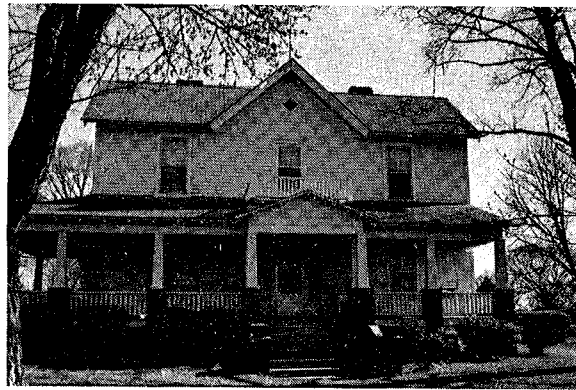
SITE NAME: Hayward Simpson House LOCATION: Haw River AGE: 1894 BUILDING MATERIAL: Frame CHIMNEY: Brick
