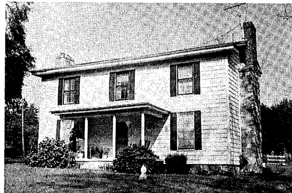
SITE NAME: Allen-Hester House LOCATION: Pleasant Grove AGE: c. 1865 FLOOR PLAN: 2A BUILDING MATERIAL: Frame CHIMNEY: Stone, Brick
