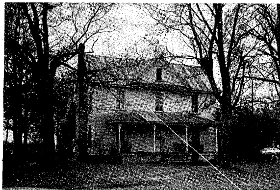
SITE NAME: J. W. Hadley House LOCATION: Newlin AGE: c. 1885 FLOOR PLAN: 6 BUILDING MATERIAL: Frame CHIMNEY: Stone, Brick
