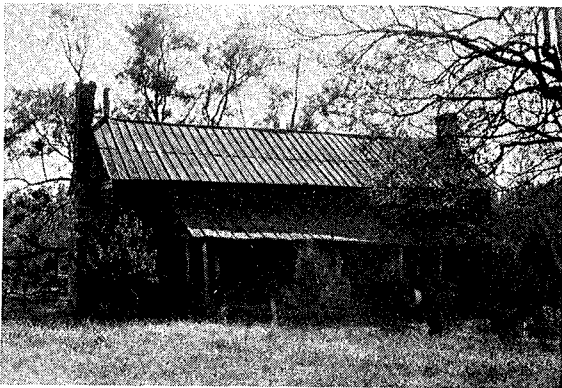
SITE NAME: Alfred Iseley House LOCATION: Morton AGE: 1852 FLOOR PLAN: 2, Dogtrot BUILDING MATERIAL: Log CHIMNEY: Stone, Brick
