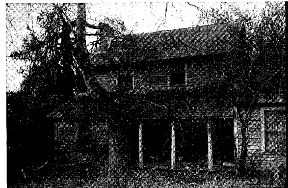
SITE NAME: William Wright House LOCATION: Patterson AGE: (?) FLOOR PLAN: 2A BUILDING MATERIAL: Log CHIMNEY: Stone, Brick
