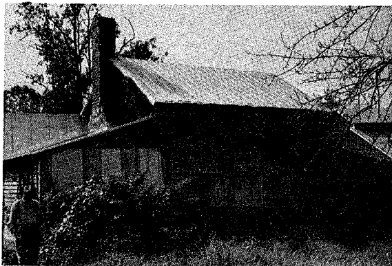
SITE NAME: William Lineberry House LOCATION: Pleasant Grove AGE: 1887 FLOOR PLAN: 1 BUILDING MATERIAL: Log CHIMNEY: Stone, Brick
