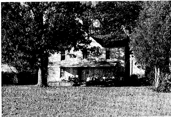
SITE NAME: J. A. Riddle House LOCATION: Newlin AGE: c. 1880 FLOOR PLAN: 6 BUILDING MATERIAL: Frame CHIMNEY: Stone, Brick
