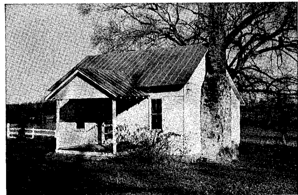
SITE NAME: Ward Mill House LOCATION: Patterson AGE: c. 1885 FLOOR PLAN: 2 BUILDING MATERIAL: Frame CHIMNEY: Stone, Brick
