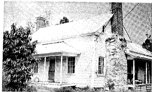
SITE NAME: John Long House LOCATION: Pleasant Grove AGE: c. 1850 FLOOR PLAN: 2A BUILDING MATERIAL: Frame CHIMNEY: Stone, Brick
