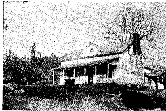
SITE NAME: Ben Sutton House LOCATION: Morton AGE: c. 1885 FLOOR PLAN: 2 BUILDING MATERIAL: Frame CHIMNEY: Stone, Brick
