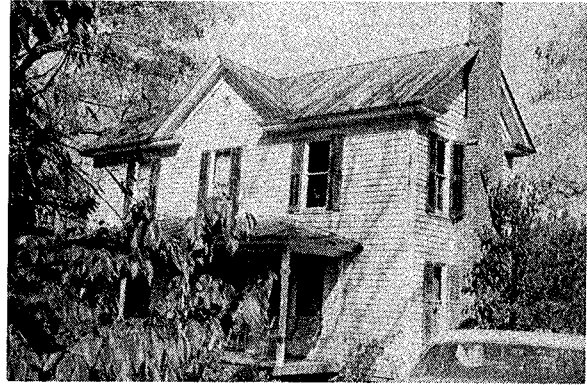
SITE NAME: A. J. Albright House LOCATION: Coble AGE: c. 1850, c. 1880 FLOOR PLAN: 1, 2 BUILDING MATERIAL: Frame CHIMNEY: Brick
