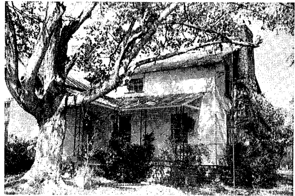
SITE NAME: Will Cooper House LOCATION: Albright AGE: (?) Pre 1893; Remodeled 1920 FLOOR PLAN: 2 BUILDING MATERIAL: Log CHIMNEY: Stone, Brick
