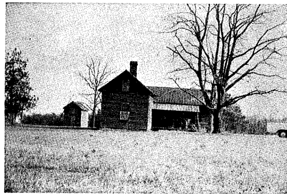
SITE NAME: J. T. Moore House LOCATION: Morton AGE: c. 1885 FLOOR PLAN: 1 BUILDING MATERIAL: Log CHIMNEY: Stone, Brick
