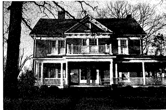
SITE NAME: L. E. Atwater House LOCATION: Burlington AGE: 1890 BUILDING MATERIAL: Frame, Brick CHIMNEY: Brick
