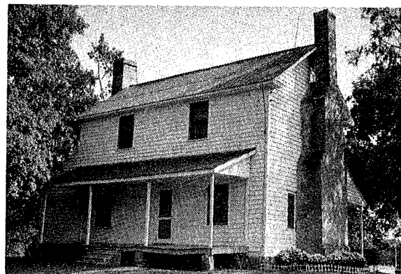
SITE NAME: J. M. Hurdle House LOCATION: Faucette AGE: c. 1840 FLOOR PLAN: 2 BUILDING MATERIAL: Frame CHIMNEY: Stone, Brick
