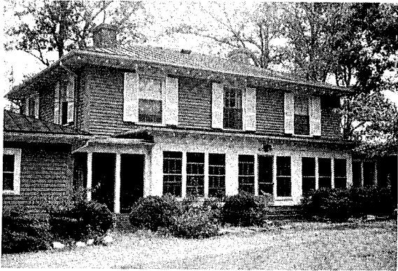
SITE NAME: B. Frank Mebane House LOCATION: Melville AGE: 1855 FLOOR PLAN: 4 BUILDING MATERIAL: Frame CHIMNEY: Brick
