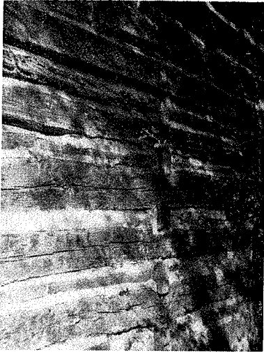
Interior log partition extends to exterior
