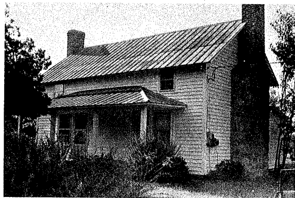
SITE NAME: J. M. Story House LOCATION: Morton AGE: c. 1850 FLOOR PLAN: 2 BUILDING MATERIAL: Log CHIMNEY: Stone, Brick
