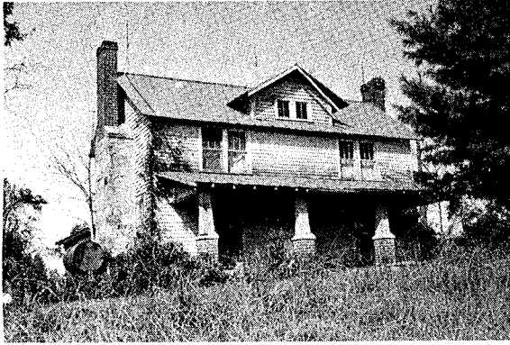
SITE NAME: Widow Gilliam House LOCATION: Morton AGE: (?) FLOOR PLAN: 2A BUILDING MATERIAL: Frame CHIMNEY: Stone, Brick
