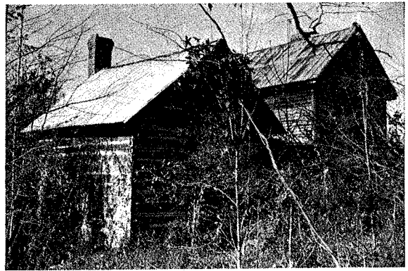
SITE NAME: J. Benjamin Thompson House LOCATION: Thompson AGE: (?) c. 1850; c. 1900 addition FLOOR PLAN: 1; 2 BUILDING MATERIAL: Log; Frame CHIMNEY: Stone, Brick; Brick
