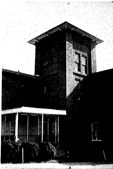
SITE NAME: Hopedale Cotton Mill LOCATION: Faucette AGE: 1869 BUILDING MATERIAL: Brick CHIMNEY: Brick
