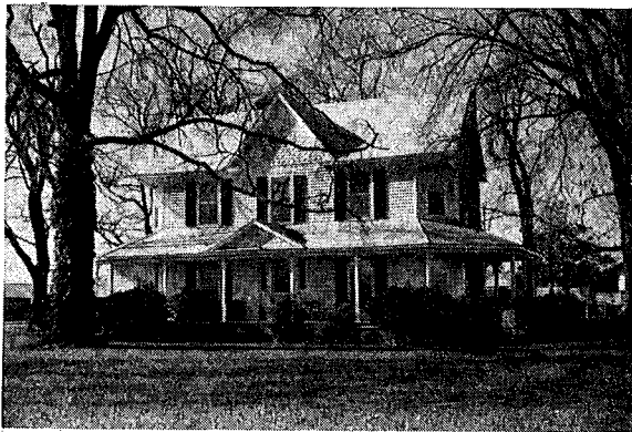
SITE NAME: S. L. Bradshaw House LOCATION: Thompson AGE: 1910 FLOOR PLAN: 6 BUILDING MATERIAL: Frame CHIMNEY: Brick
