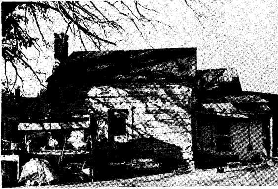
SITE NAME: Arch Crabtree House LOCATION: Albright AGE: c. 1850 FLOOR PLAN: 1 BUILDING MATERIAL: Log CHIMNEY: Stone, Brick
