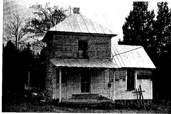
SITE NAME: Snow Camp Telephone Exchange LOCATION: Newlin AGE: (?) c. 1900 BUILDING MATERIAL: Frame CHIMNEY: Stone
