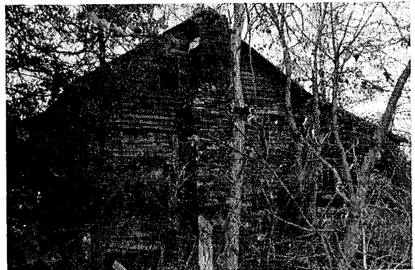
SITE NAME: B. Holt House LOCATION: Albright AGE: c. 1870 FLOOR PLAN: 2 BUILDING MATERIAL: Log CHIMNEY: Stone, Brick
