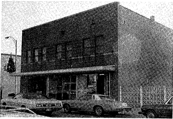
SITE NAME: Rauhut Building LOCATION: Burlington AGE: Pre 1886 BUILDING MATERIAL: Brick CHIMNEY: Brick
