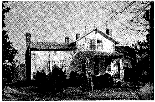
SITE NAME: Natty Woody Site, S.E. Woody House LOCATION: Newlin AGE: 1891 FLOOR PLAN: 2A BUILDING MATERIAL: Frame CHIMNEY: Stone, Brick
