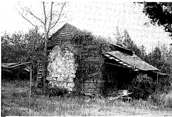
SITE NAME: Bivins Log House LOCATION: Newlin AGE: c. 1840 FLOOR PLAN: 2 BUILDING MATERIAL: Log CHIMNEY: Stone
