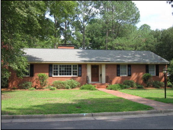
1307 Summit Street, ca. 1950s This Ranch house nicely illustrates the typical horizontal Ranch form and minimally applied Colonial Revival details, such as fluted entry pilasters a divided-light window sash.
