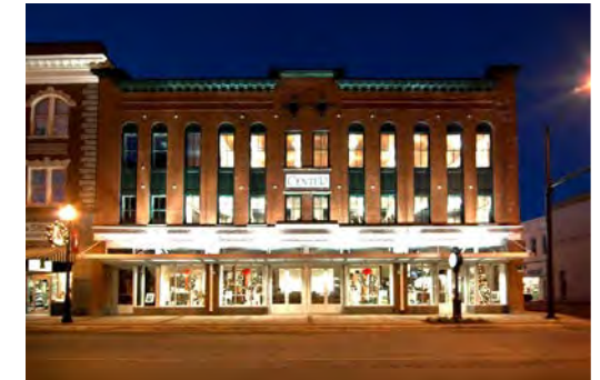
Lowry-Chesson Bldg. Elizabeth City / Pasquotank Co.
